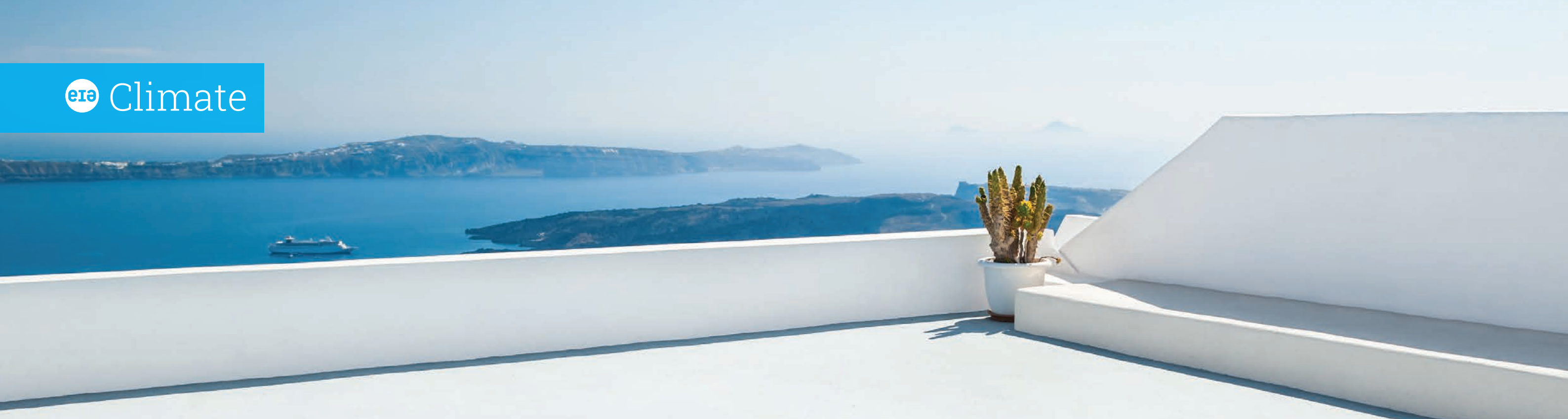
Above: A cool roof painted white to reflect sunlight and absorb less heat.
