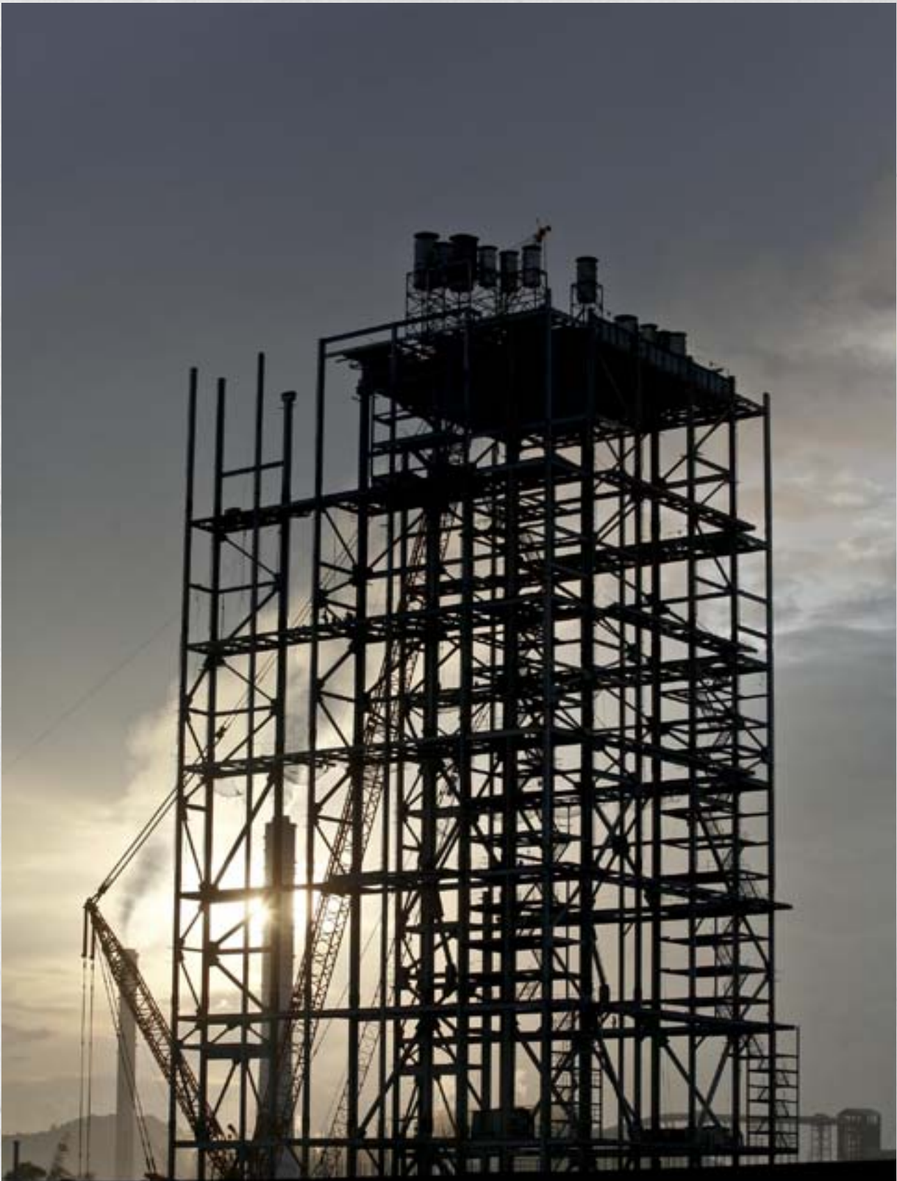
Image: "Anpara-D", a new wing of the Anpara thermal power plant under construction.
