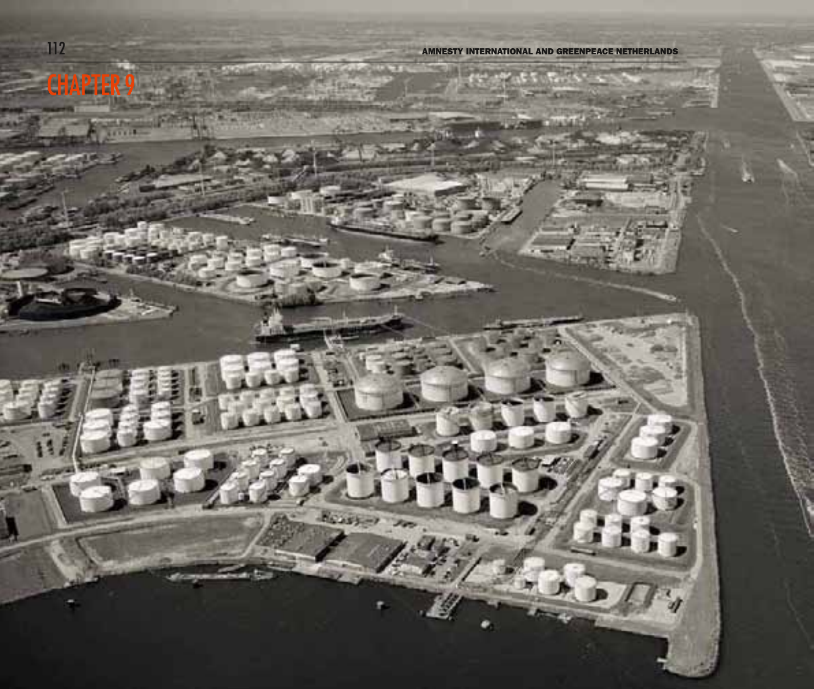
Aerial view of the Port of Amsterdam © ANP/YOUR CAPTAIN LUCHTFOTOGRAFIE
