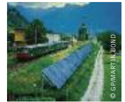
image 100 KW PV GENERATING PLANT NEAR BELLINZONA-LOCARNO RAILWAY LINE. GORDOLA, SWITZERLAND.
