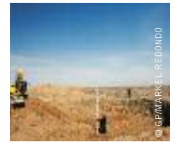
image AN EXCAVATOR DIGS A HOLE AT GUAZHOU WIND FARM CONSTRUCTION SITE, CHINA, WHERE IT IS PLANNED TO BUILD 134 WINDMILLS.
