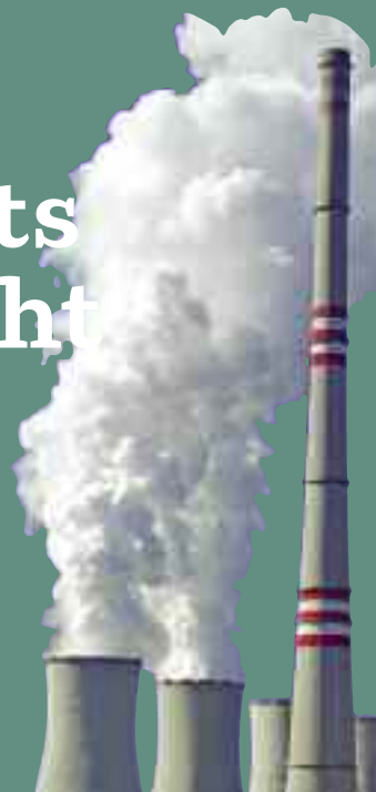
image COAL FIRED POWER PLANT. © F. FOX/DREAMSTIME
