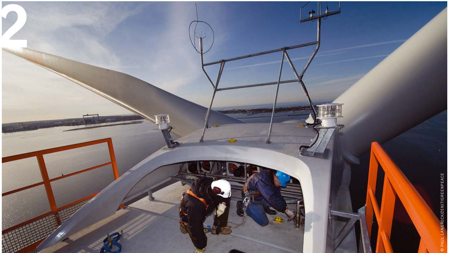
image TWO TECHNICIANS WORKING INSIDE THE TURBINE OF TEST WINDMILL N90 2500, BUILT BY THE GERMAN COMPANY NORDEX, IN THE HARBOUR OF ROSTOCK. THIS WINDMILL PRODUCES 2,5 MEGA WATT AND IS TESTED UNDER OFFSHORE CONDITIONS. AT LEAST 10 FACILITIES OF THIS TYPE WILL BE ERECTED 20 KM OFF THE ISLAND DARSS IN THE BALTIC SEA BY 2007. TWO TECHNICIANS WORKING INSIDE THE TURBINE.
