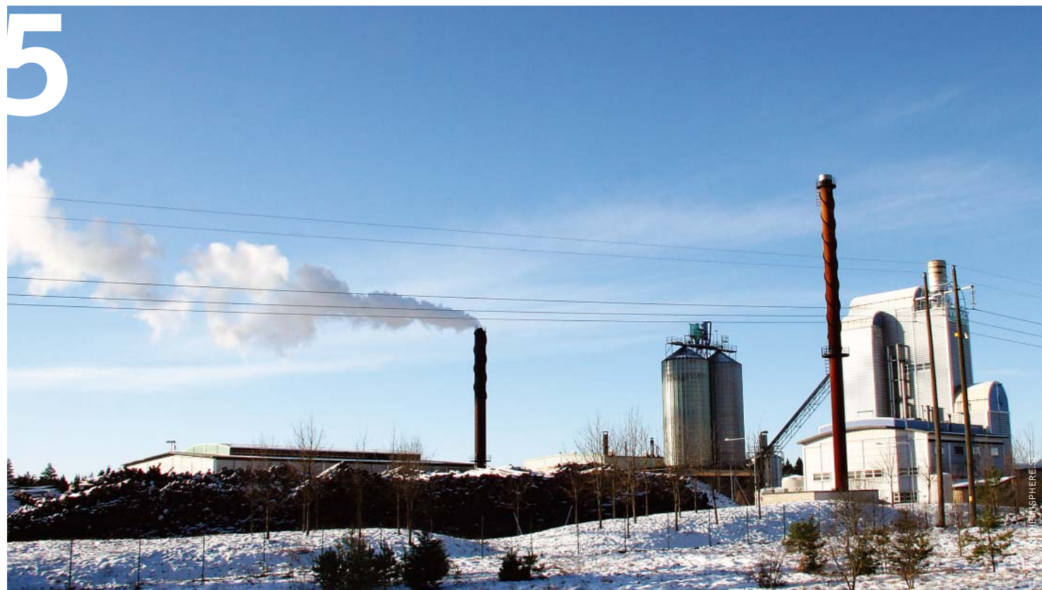
image BIOMASS ENERGY PLANT NEAR VARNAMO, SWEDEN.
