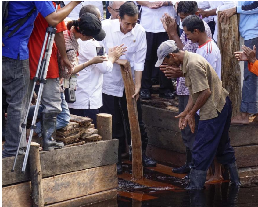
27 November 2014, Sungai Tohor, Riau: Indonesian President Joko Widodo joins members of the Sungai Tohor community in damming a canal draining the surrounding peatland. ©Rante/Greenpeace
