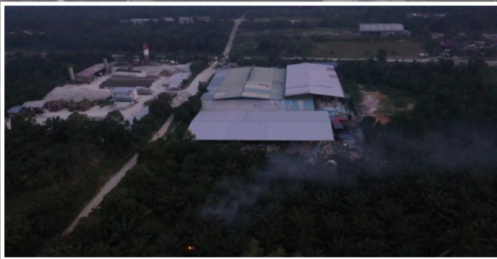
Plastic recycling facility in Kapar, Klang. The picture shows smoke from burning mixed waste, which includes plastics.
