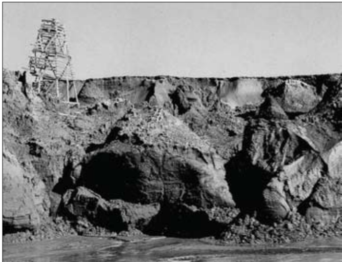
Fig. 7. The Vankin navigational sign slips vertically, later to be destroyed. Location: The southern coast of the Bolshoy Lyahovsky Island in the Eastern Siberian Sea. Photo by M. Grigoryev.
