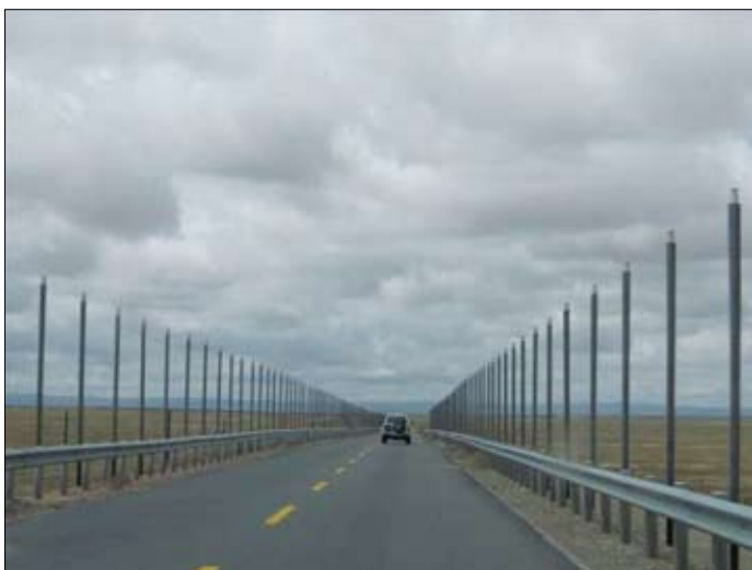
Fig. 23. Examples of line structures in conditions of glaciers on the Tibet plateau (in China) where construction techniques have been adapted to consider the impacts of climate change. On the left: thermo-stabilization of railway and road embankments has been undertaken with the aid of cooling thermosyphons. On the right: a set of cooling ventilation channels placed in the embankment of a road. On the lower right: a vehicle road built upon unstable soil using a flyover principle with deepened supports. Photo by N. I. Shiklomanov.
