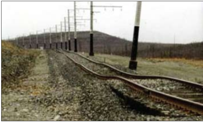
Fig. 22. On the left: A section of the Baikal-Amur Mainline affected by deformation due to non-uniform subsidence and soil-heave. On the right: this deformation of abandoned military facilities in the low part of the Yenisey river occurred due to non-uniform thawing of underground ice. Photo by D. S. Drozdov.
