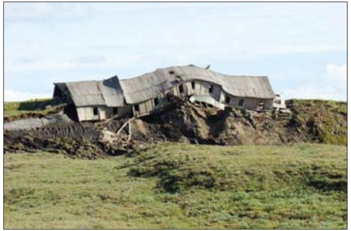
Fig. 22. On the left: A section of the Baikal-Amur Mainline affected by deformation due to non-uniform subsidence and soil-heave. On the right: this deformation of abandoned military facilities in the low part of the Yenisey river occurred due to non-uniform thawing of underground ice. Photo by D. S. Drozdov.
