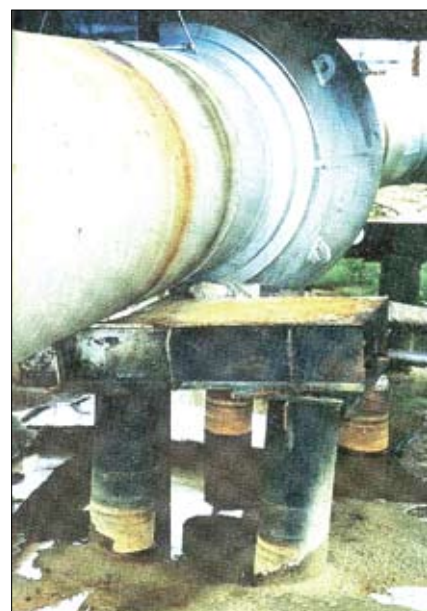
Fig. 24. On the left: supports for an Alaskan pipeline using thermosyphons. Photo by N.I.Shikllomanov. On the right: deformation of a pipeline support in Western Siberia. Photo from (Garagulya, Ershov, 2000)
