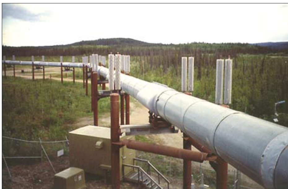
Fig. 24. On the left: supports for an Alaskan pipeline using thermosyphons. Photo by N.I.Shikllomanov. On the right: deformation of a pipeline support in Western Siberia. Photo from (Garagulya, Ershov, 2000)
