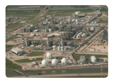
This photo shows the Oyster Creek complex, which houses multiple chlorine facilities. Chlorine is manufactured here and used to produce precursors to PVC and other products.
