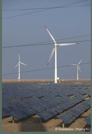
Dafeng Power Station is Chinas largest solar photovoltaic-wind hybrid power station, with 220MW of grid-connected capacity, of which 20 MW is solar PV. Located in Yancheng, Jiangsu province, it came into operation on December 31, 2010 and has 1,100 annual utilization hours.
