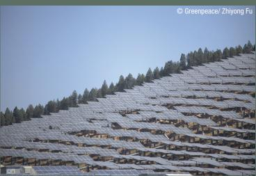
The Xuzhou Solar Photovoltaic Power Station was connected to the grid on December 30, 2009. With an installed capacity of 20MW, it has 1,300 annual utilization hours and can generate about 26 million Kw-h of electricity each year equivalent to savings of 7,900 tons of coal and 21,000 tons of carbon dioxide emissions.
