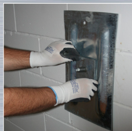
7. Install Wall Plate and Tighten System
