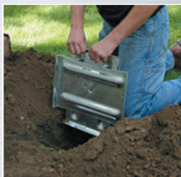
6. Attach Outside Earth Anchor
