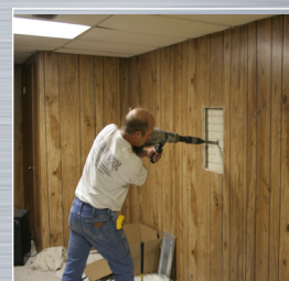
4. Drill Hole in Basement Wall
