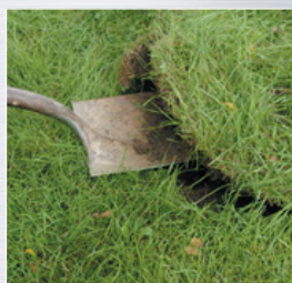
2. Remove and Save Sod
