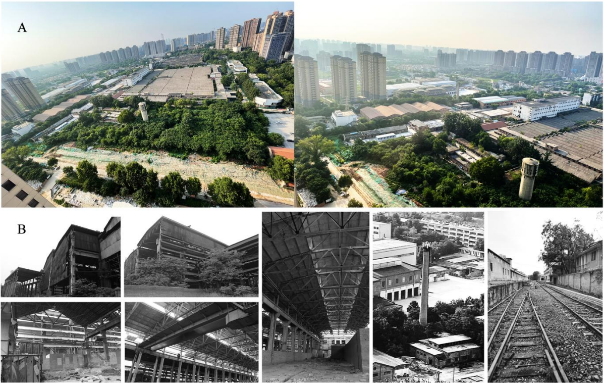
Fig 7. Site spatial-physical status and industrial heritage construction.
