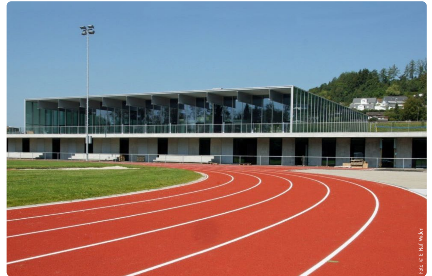
Sportzentrum Burkertsmatt in Widen
