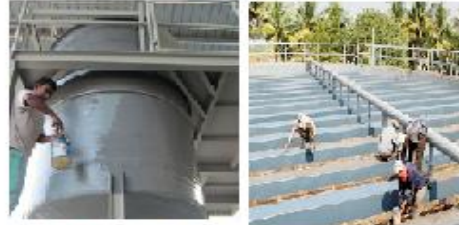
FRP LINING / COATING JOBS
