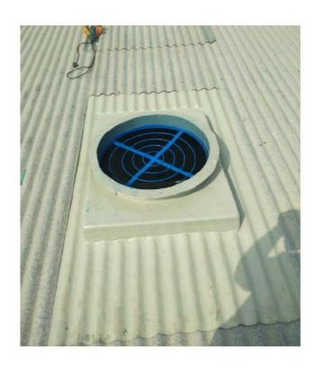
2. MOTOR ATTACHMENT - IT IS BOLTED WITH THE BASE PLATE. DESIGNED IN SUCH A WAY THAT IF ANY MAINTENANCE OR CLEANING OF EXHAUST FAN IN FUTURE REQUIRED YOU CAN EASY REMOVE AND BRING THE FAN DOWN WITHOUT REMOVING BASE PLATE.
