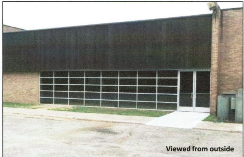
New exterior windows &amp; doors
