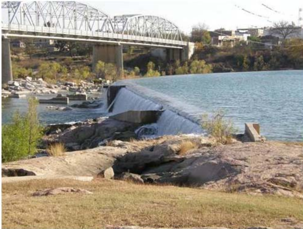
This is a photo of Roy Inks Bridge and Dam in Llano Texas. The bridge was built by Austin Bridge Company in the 1930's.
