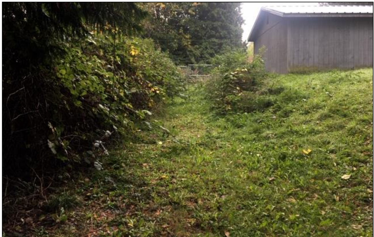
Photo 2. Western overview of the pumphouse APE.
