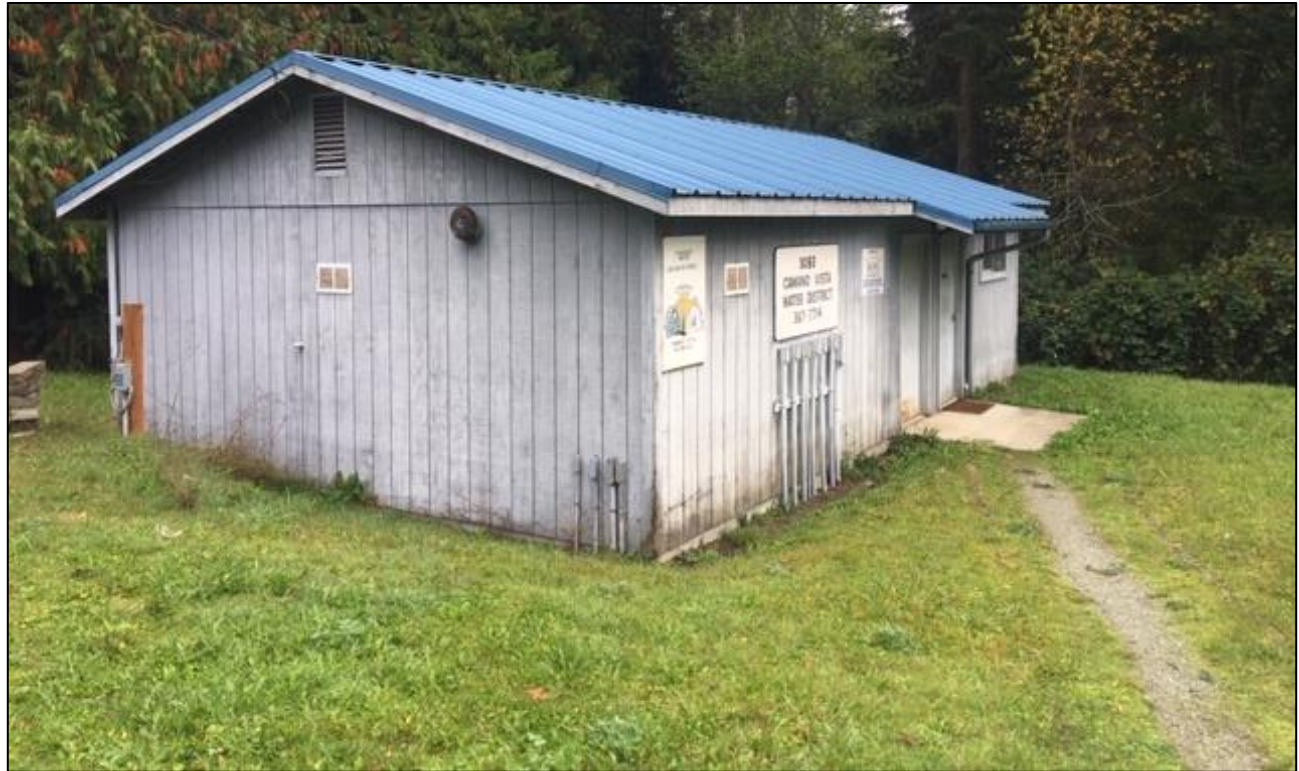
Photo 1. Northern overview of the pumphouse APE.
