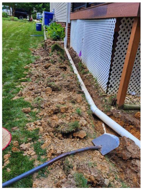
In this example, roof runoff from the downspout is diverted underground to the excavated rain garden area and is connected to a pop up emitter which allows water to discharge into the rain garden. The berm retains the water allowing it to infiltrate instead of running off, causing erosion.
