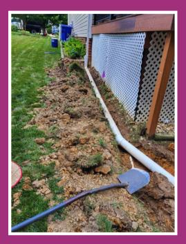
In this example, roof runoff from the downspout is diverted underground to the excavated rain garden area and is connected to a pop up emitter which allows water to discharge into the rain garden. The berm retains the water allowing it to infiltrate instead of running off, causing erosion.
