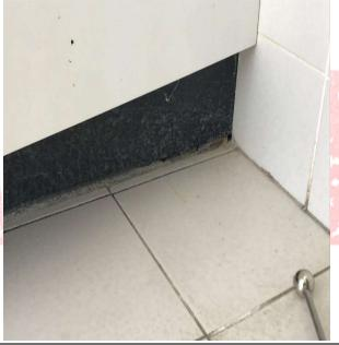
Ensuite has areas of drumming tiles which is consistent with the tiles separating from the surface behind them,
