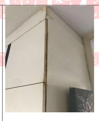
B2 BIR has dropped due to water damage and rote in its base causing it to crack along the ceiling,
