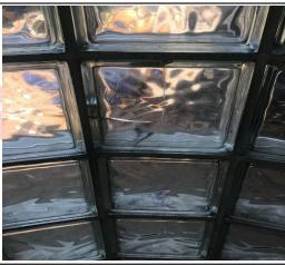
Ground level outside of B2 sliding door is higher than the floor level, Glazing seals have retracted and require replacing, Sealant around glass brick has retracted and cracked on the outside in multiple places, Multiple cracked glass bricks in both the Bathroom / Laundry and Ensuite,
