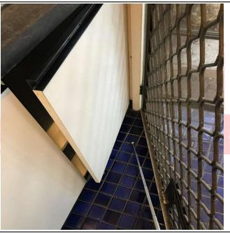
Kitchen has areas of drumming tiles which is consistent with the tiles separating from the surface behind them,
