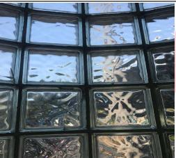
Multiple cracked glass bricks in both the Bathroom / Laundry and Ensuite,
