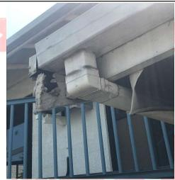
Timber barge has obvious signs of decay and requires replacing in multiple areas,
