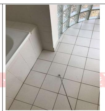
Ensuite has areas of drumming tiles which is consistent with the tiles separating from the surface behind them,
