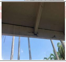
Condensation pipe from Split system needs to be diverted away from house,
