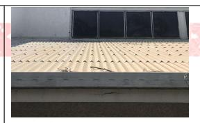
Gutters have a build leaf letter and require cleaning, Gutters have a build leaf letter and require cleaning, Roof cladding appears to be in good condition for the age of the building, Fixings will require replacing in the near future as they have begun to rust, Gutters have a build leaf letter and require cleaning,
