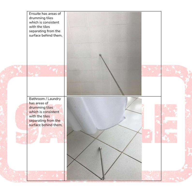
Bathroom / Laundry floor tiles in shower has areas of drumming which is consistent with the tiles separating from the surface behind them, these tiles have also been replaced and are not consistent with the rest of the room,
