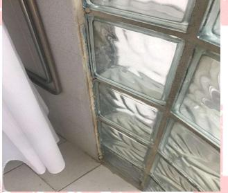
Bathroom / Laundry join between glass bricks and wall requires sealing, this area is exposed to the shower and vitally important,
