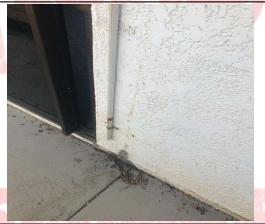
Security camera has become detached from the wall. Rust has started to form on the carport purlins. Paving at the back door is lower than the drain resulting in water pooling, Rust has started in the back door jamb leading into kitchen,
