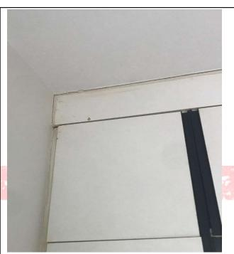
B2 BIR has dropped due to water damage and rote in its base causing it to crack along the ceiling,
