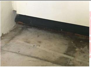
B2 BIR has dropped due to water damage and rote in its base, causing cracks between the BIR and the ceiling, B2 BIR has dropped due to water damage and rote in its base causing it to crack along the ceiling,
