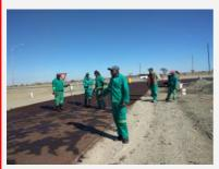
busy with road maintenance on the turn-off to Krönlein from the B1. The road was in a very bad condition and the team will be patching potholes, and sealing it with a new layer of slurry. The work is expected to be completed by 15 June 2020.
