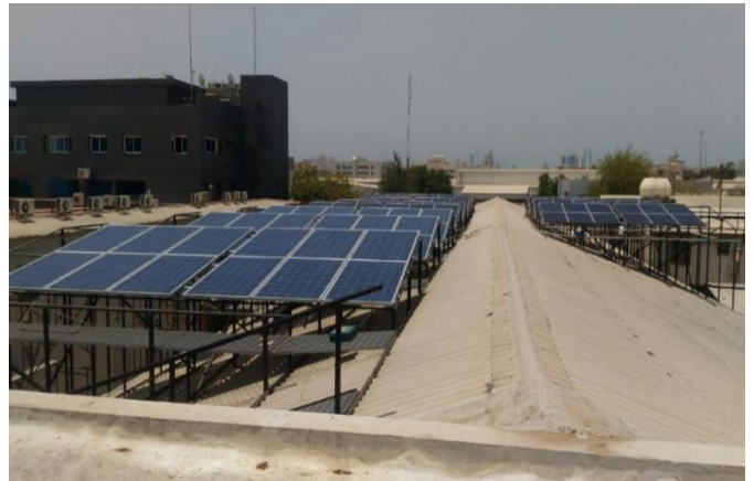
Factory Roof Top
