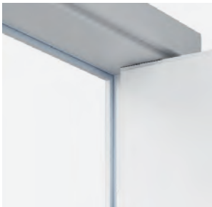
Door frame corner from hinges side
