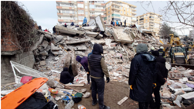
The wreckage of a collapsed building, Diyarbakir, Turkey. (Photo: VOA courtesy of Wikimedia Commons; public domain.)
