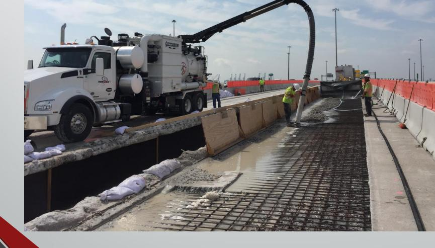
Method 1 – Fast Track Hydrodemolition & Concrete Overlays of Bridge Decks (most common)
