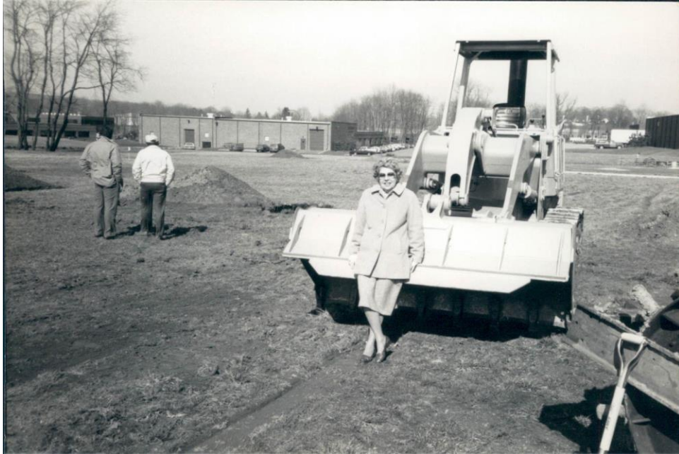
(Breaking ground for a much expanded VFTL Hq. in Exton)
