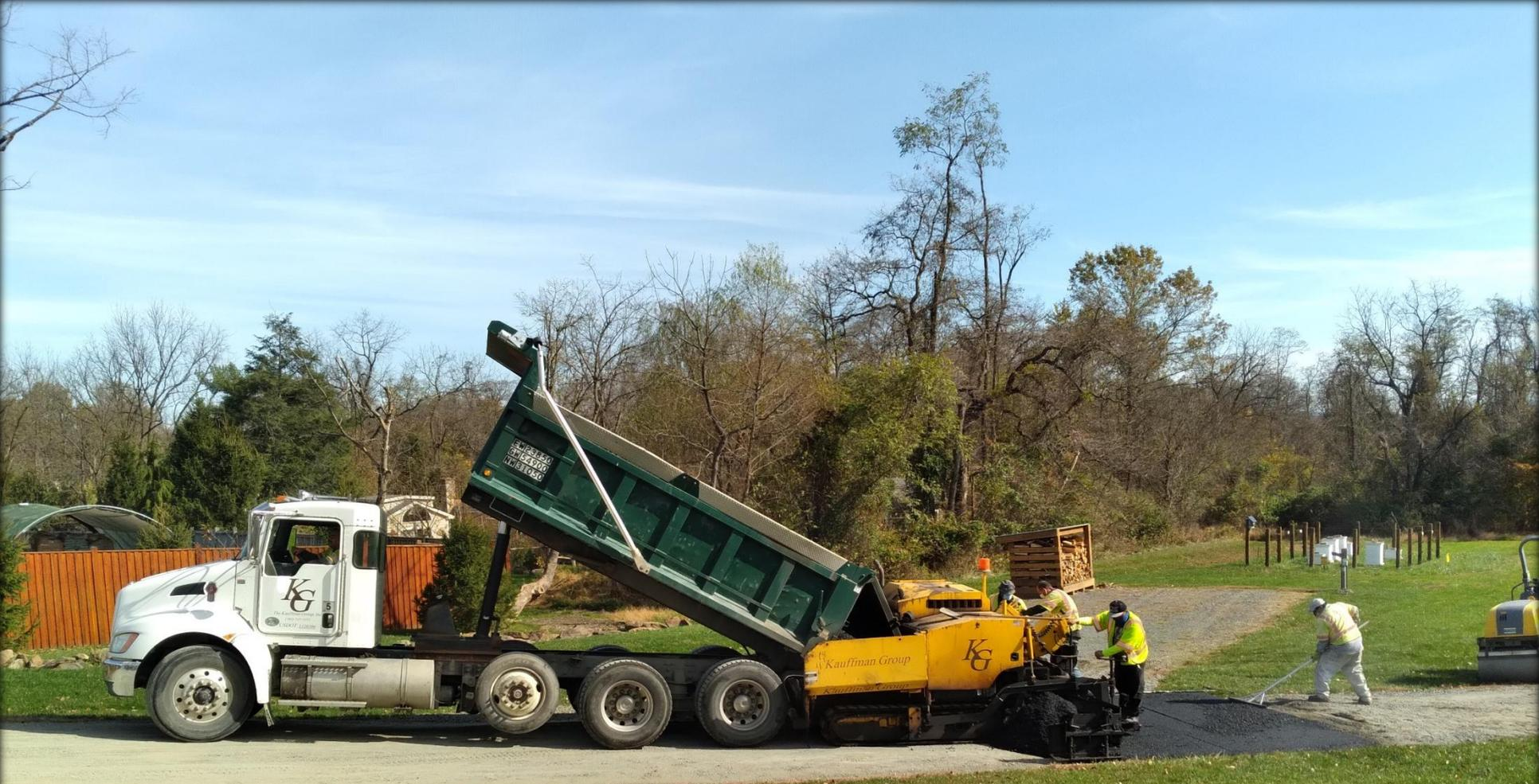
*Apply base asphalt, extending paved road surface to prevent further erosion and maintenance required on the hill area leading from the maintenance building to the barn area.*
