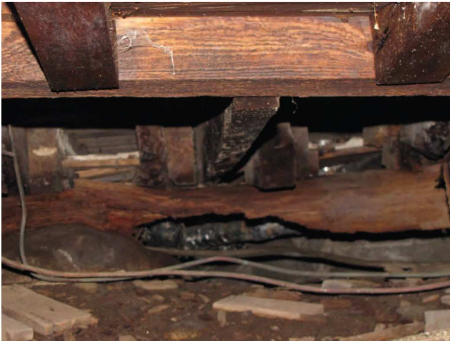
Photo 07: The southerly first floor beam in west section of the building, showing it's loss of cross-sectional depth and rotted condition, making this beam unsafe.
