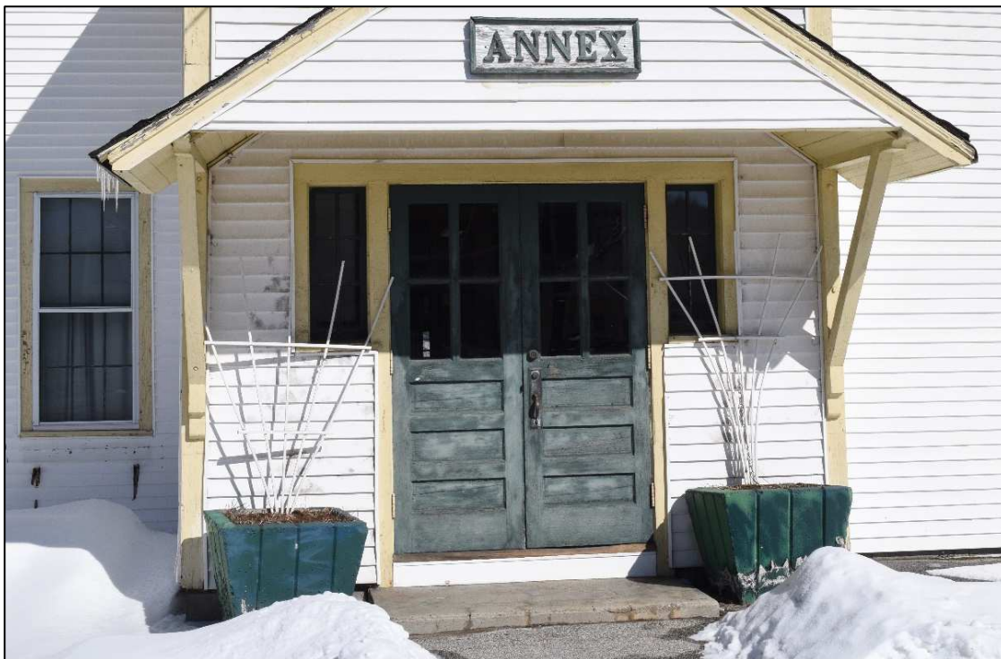
Figure III-4: Non-ADA-compliant primary entry
