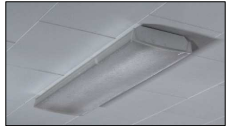
Figure III-7: Non-historic fluorescent ceiling fixture in main hall
