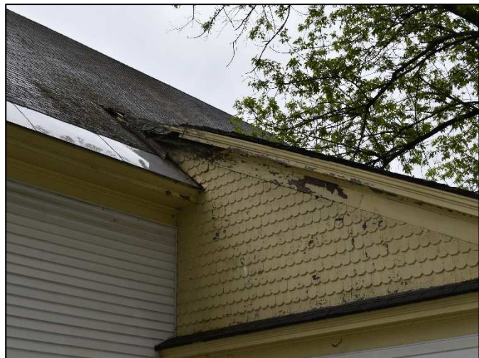
Figure III-1: Damage to roof at north side of building
