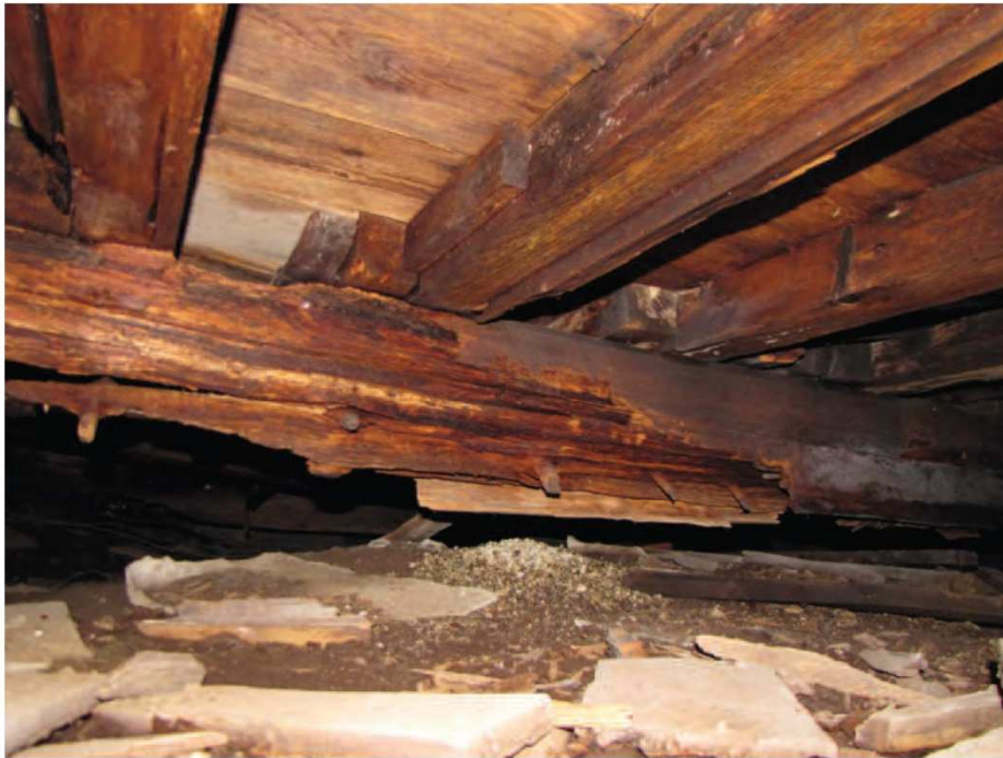
Photo 01: The northerly first floor beam in west section of the building showing it's rotted condition and loss of wood, making this beam unsafe.
