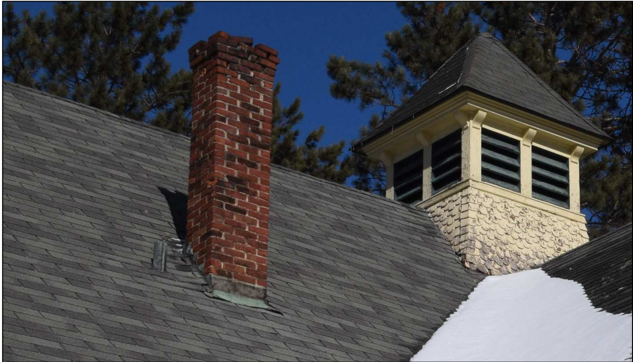
Figure III-2: Mortar deterioration at chimney
