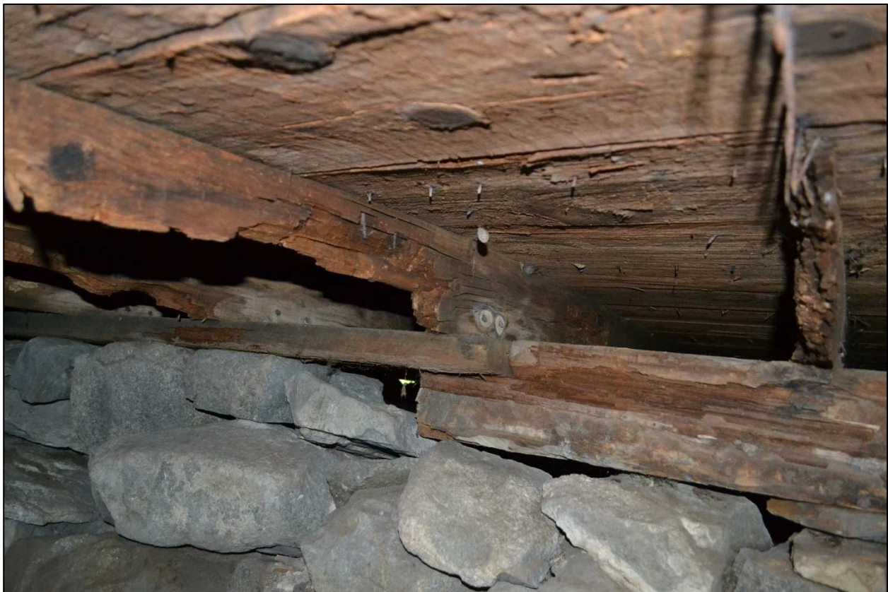
Figure III-5: Rotten floor system beneath Annex (Photograph by James L. Garvin)
