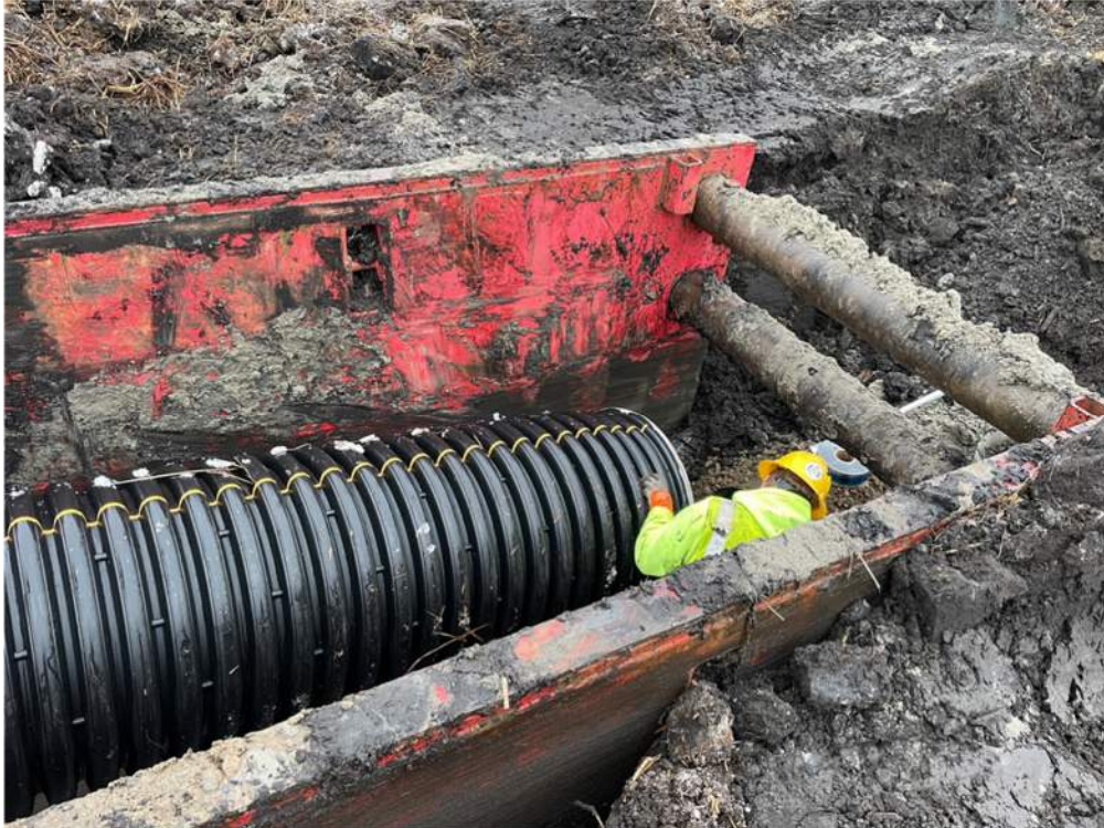
Photo #8: Installing 30" gravity flow pipe - Jan 26, 2024, 8:15 AM
