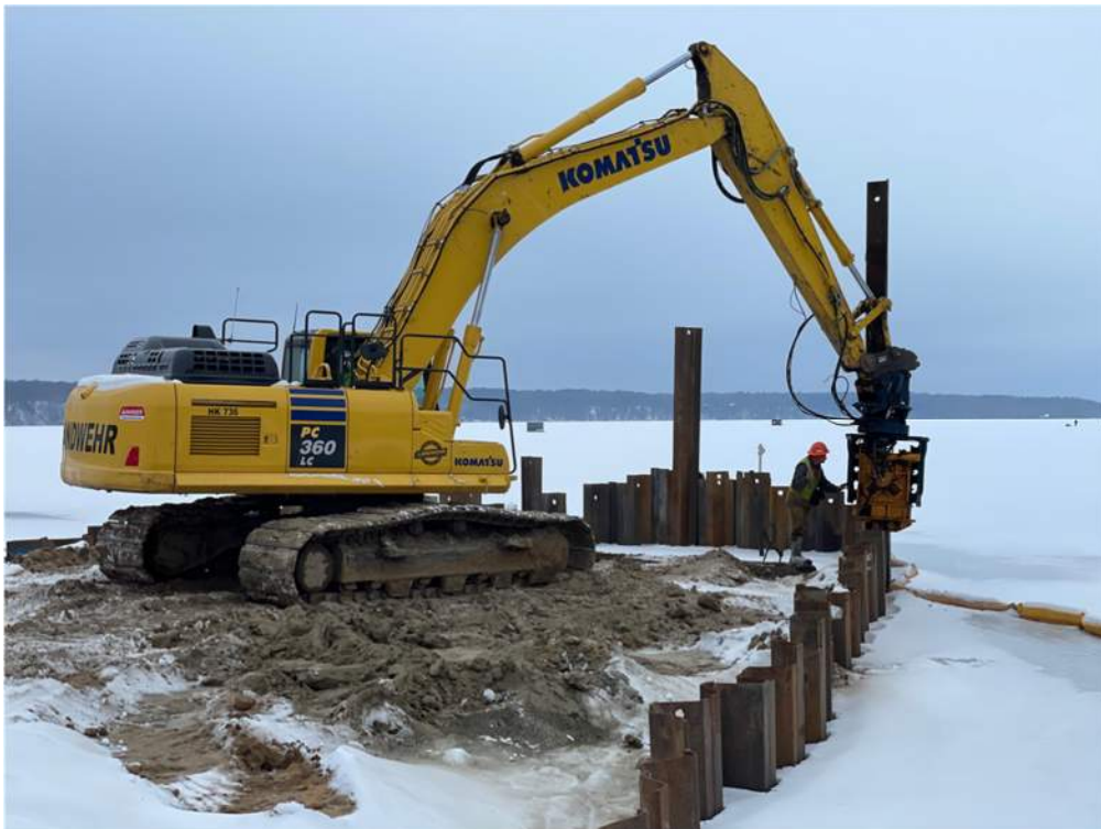
Photo #3: Removing sheeting from inlet area in the lake - Jan 23, 2024, 9:48 AM
