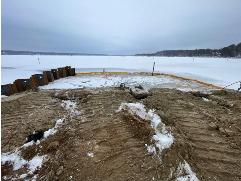
Photo #4: Sections of the sheeting wall removed - Jan 23, 2024, 12:40 PM
