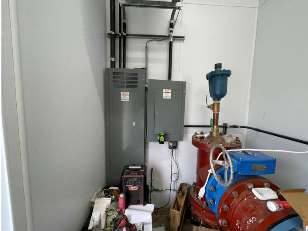
Photo #1: Interior electrical work progress - Jun 17, 2024, 3:42 PM
