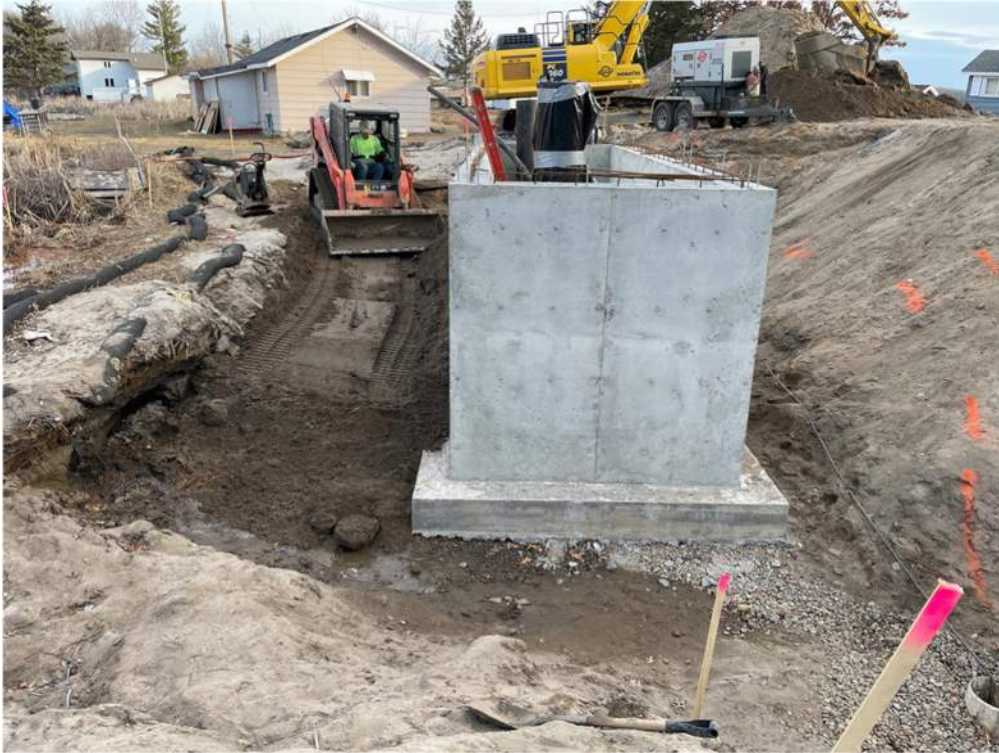
Photo #1: Backfilling around the foundation for the pump station - Feb 26, 2024, 8:21 AM
