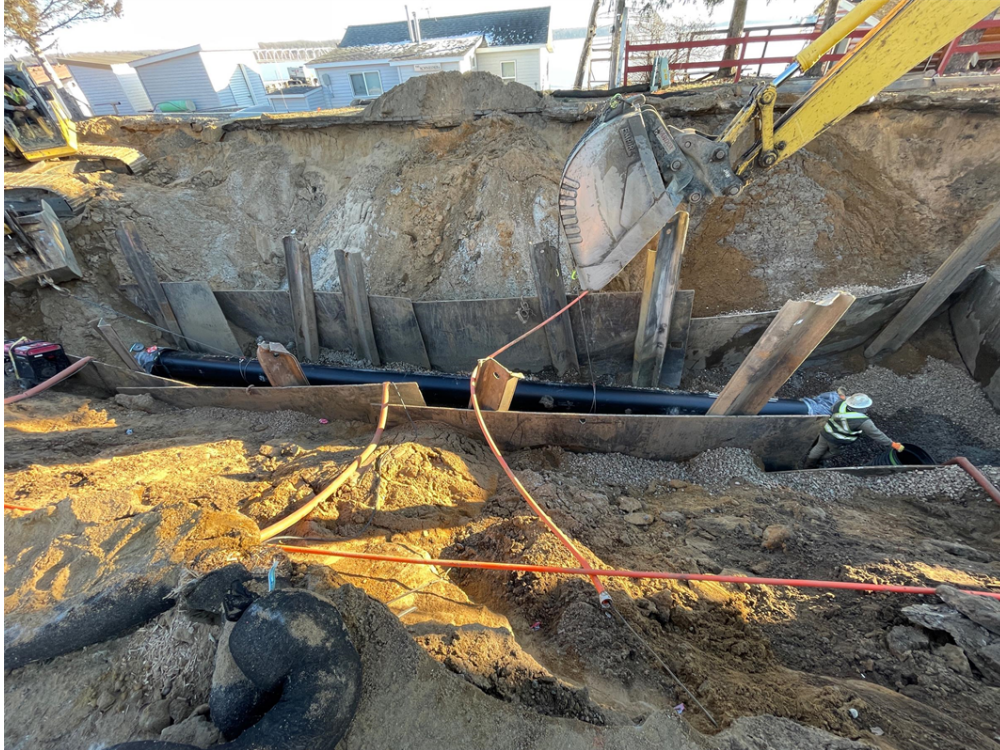
Photo #8: 50' length of 24" gravity flow pipe under Aztec Rd - Dec 14, 2023, 9:33 AM
