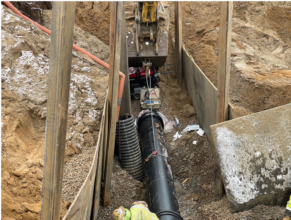
Photo #1: Fusing the coupling to the 24" gravity flow pipe - Dec 11, 2023, 11:45 AM
