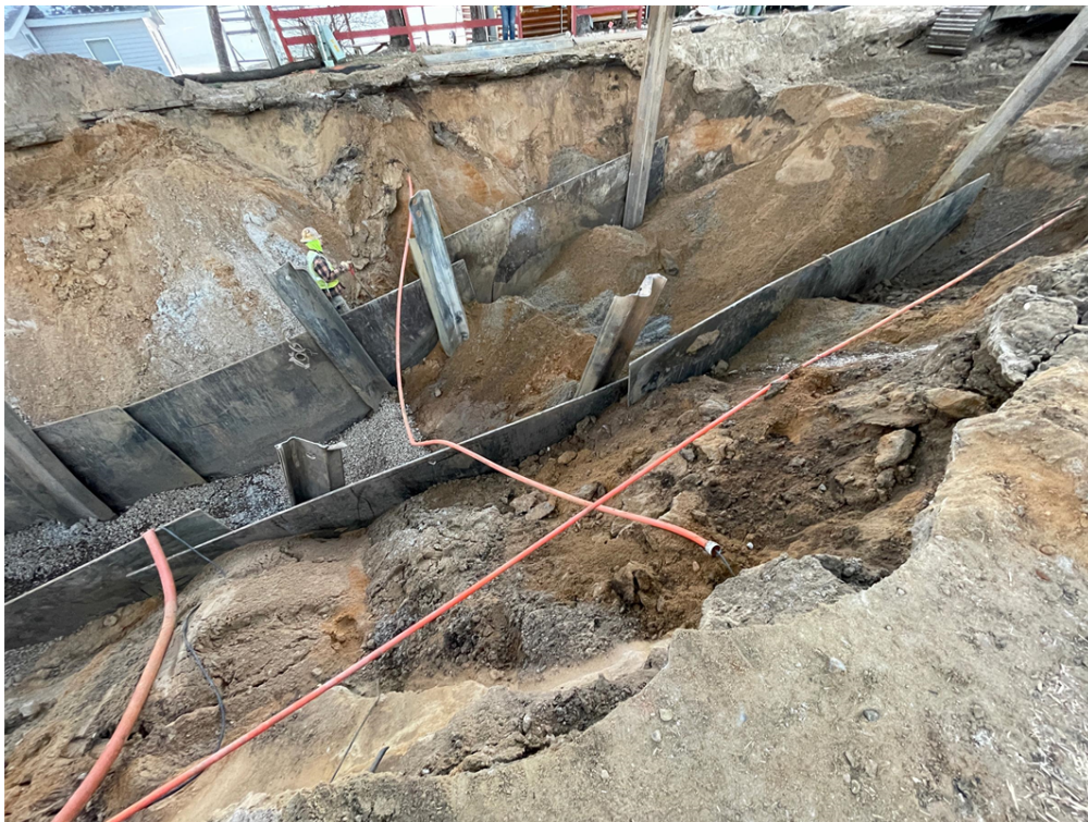
Photo #7: Fiber conduit and pipe crossing Aztec Road - Dec 14, 2023, 7:57 AM
