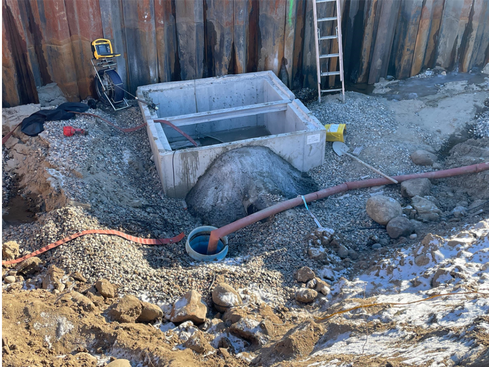
Photo #6: Concreted pipe to the inlet structure - Dec 13, 2023, 10:58 AM
