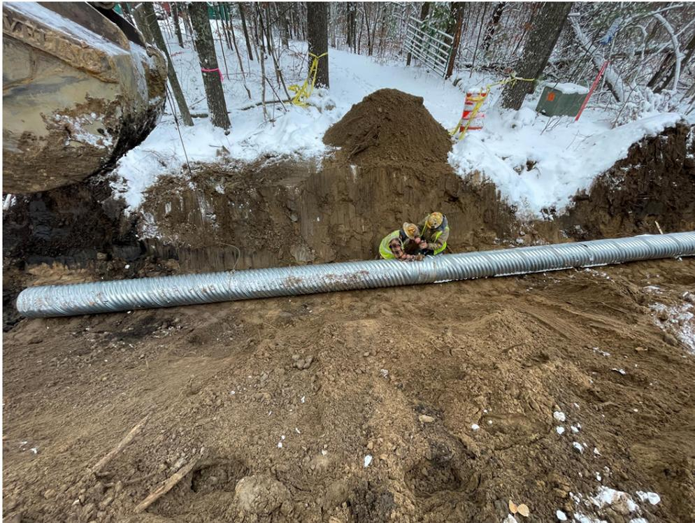
Photo #4: Installing culvert along Pulaski Road - Nov 2, 2023, 7:02 PM
