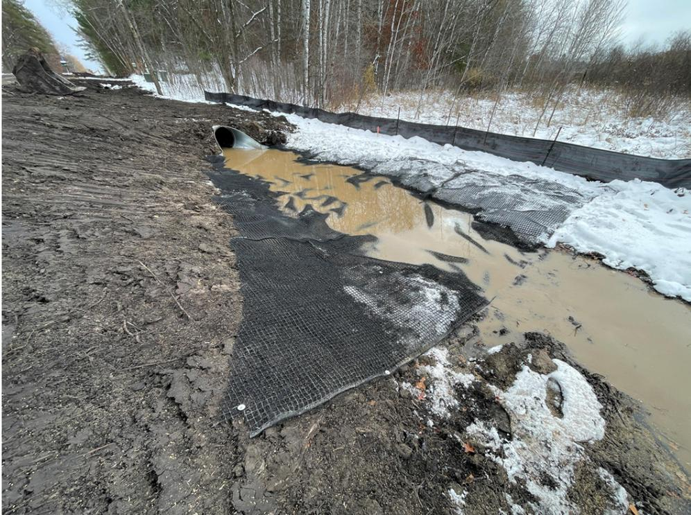
Photo #7: Turf reinforcement mat installed at the outlet end of the gravity flow pipe - Nov 2, 2023, 7:22 PM
