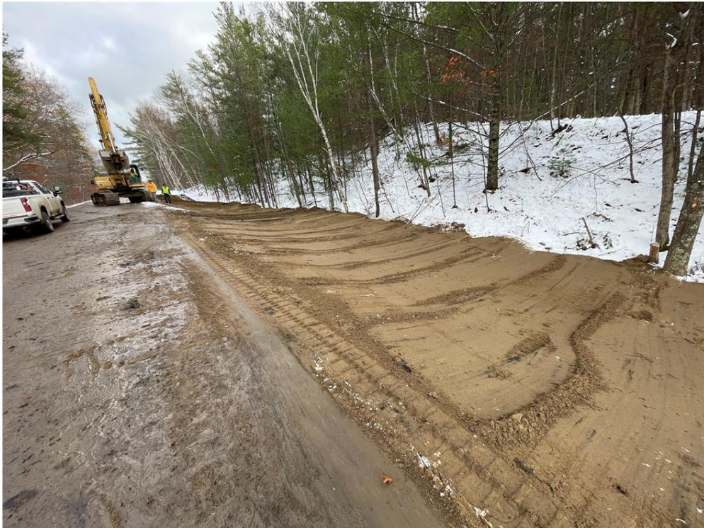
Photo #6: Restoring backfilled ditch to desired grade before adding topsoil - Nov 2, 2023, 7:06 PM
