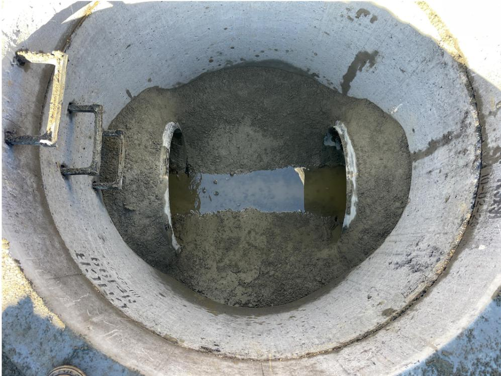
Photo #8: Concrete shelf and invert inside manhole - Nov 13, 2023, 12:30 PM
