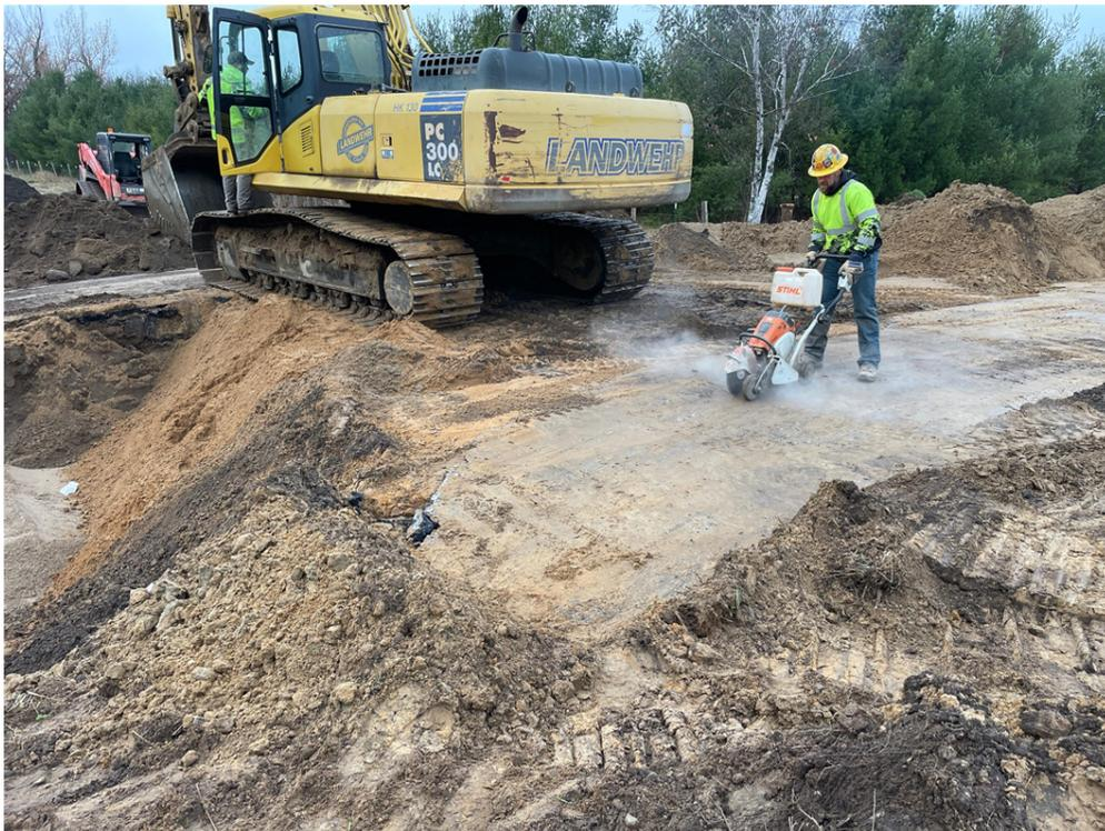
Photo #7: Cutting asphalt to remove along a straight line - Nov 8, 2023, 8:09 AM
