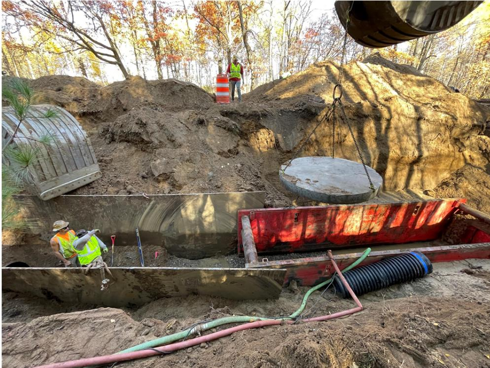
Photo #1: Installing base slab for manhole - Oct 23, 2023, 11:56 AM
