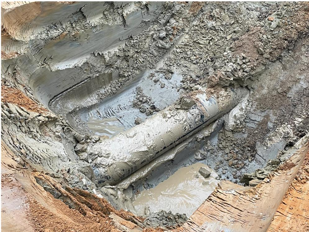
Photo #5: Bored carrier pipe going under County Road 203 - Nov 6, 2023, 7:44 AM
