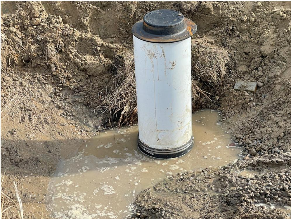
Photo #11: Tee riser structure with metal rings sealing gasket to PVC pipe - Nov 16, 2023, 11:58 AM
