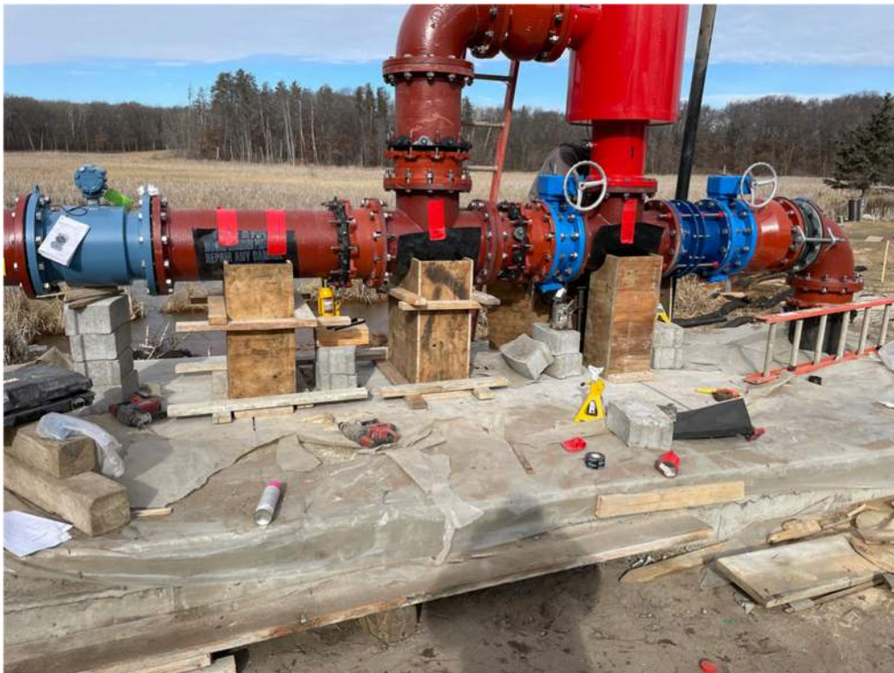
Photo #5: Forms and rebar set for the pipe supports - Mar 7, 2024, 9:54 AM
