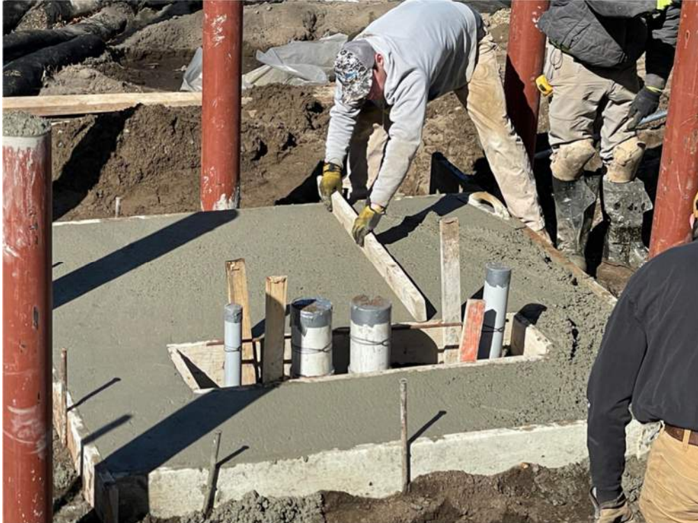
Photo #6: Leveling the concrete for the transformer pad - Mar 7, 2024, 11:24 AM
