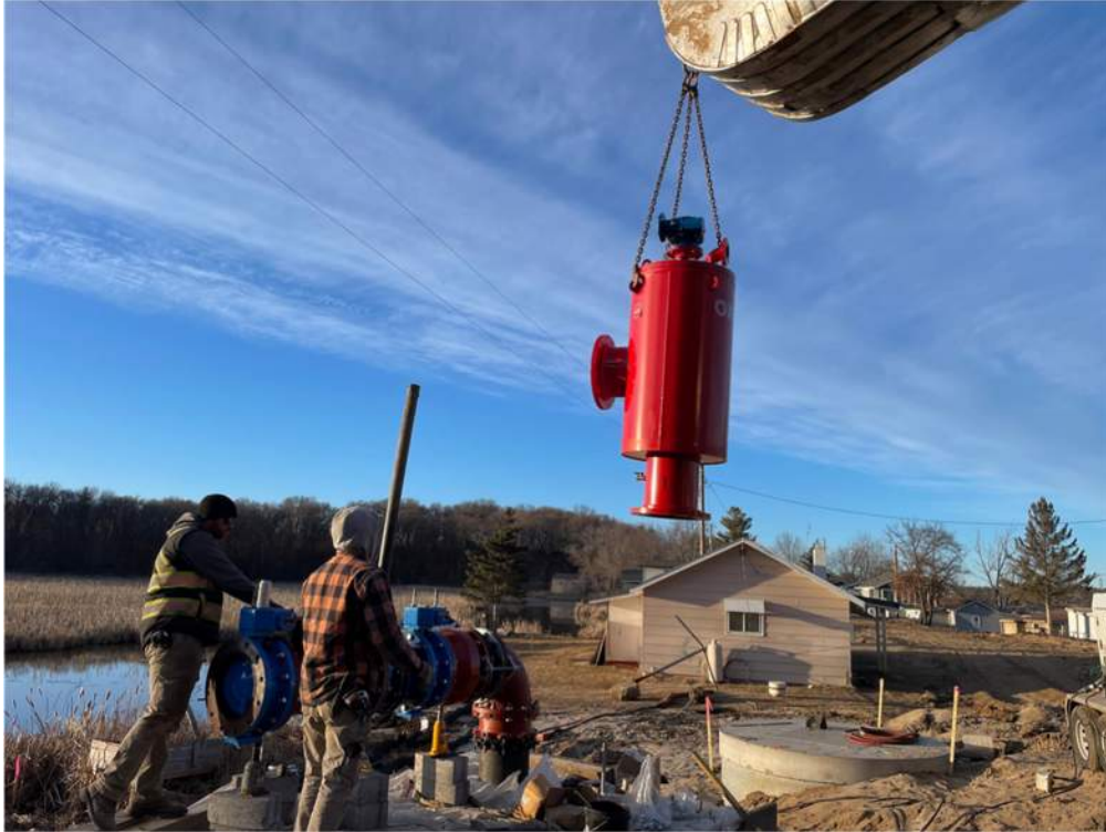
Photo #2: Lowering the Amiad filter into place - Mar 4, 2024, 5:27 PM
