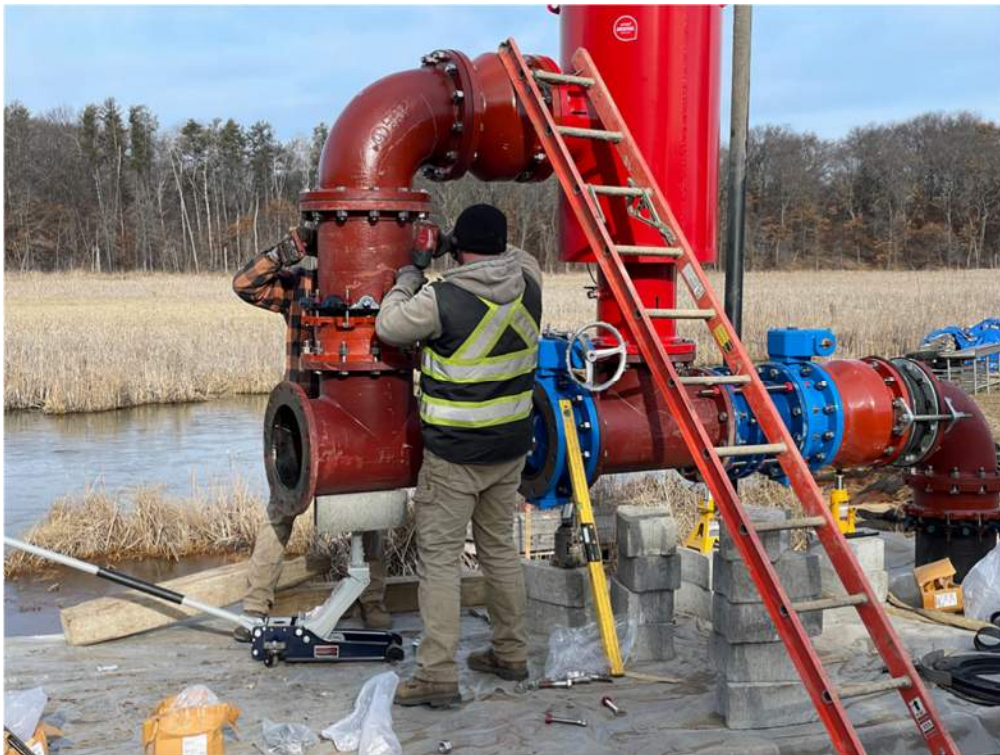
Photo #3: Installing piping and fittings for pump house - Mar 5, 2024, 9:16 AM
