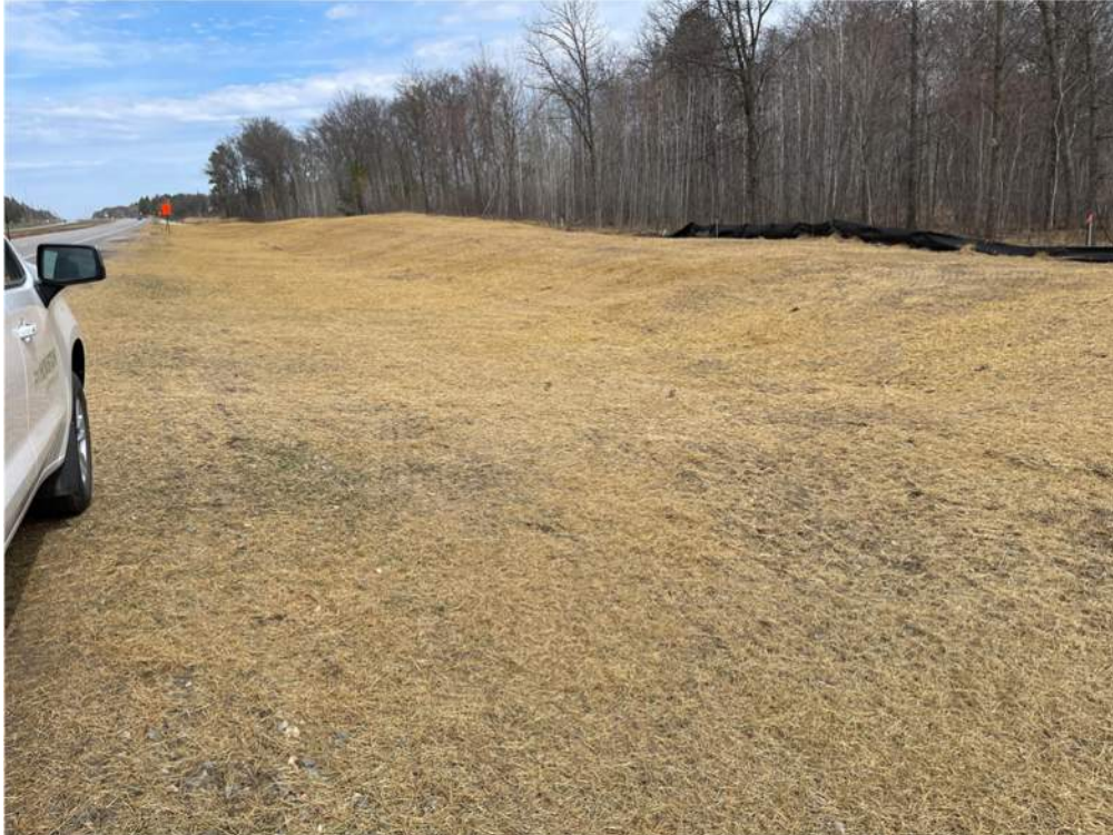
Photo #4: Ditch along Highway 10 has been seeded and mulched - Apr 15, 2024, 12:15 PM
