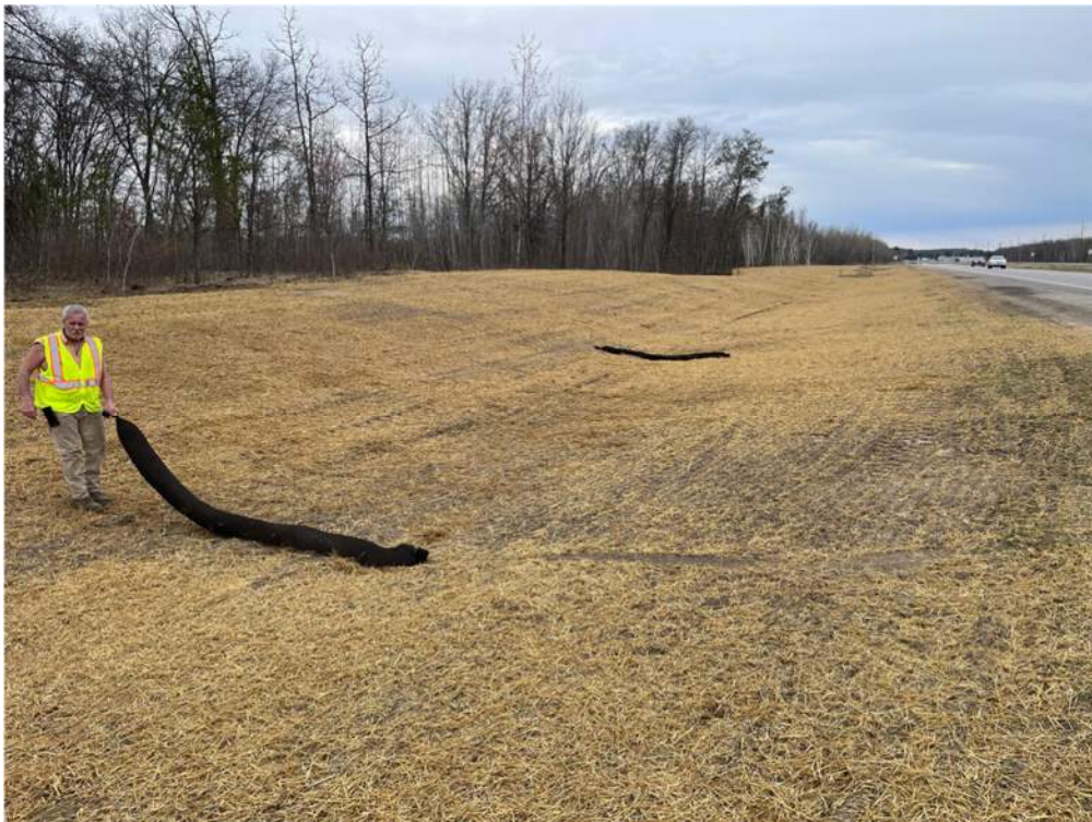
Photo #5: Installing ditch checks along Highway 10 - Apr 15, 2024, 1:00 PM
