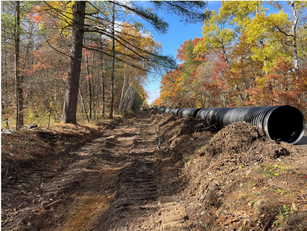
Photo #5: Ditch cleared of debris in preparation for gravity flow pipe - Oct 19, 2023, 9:29 PM
