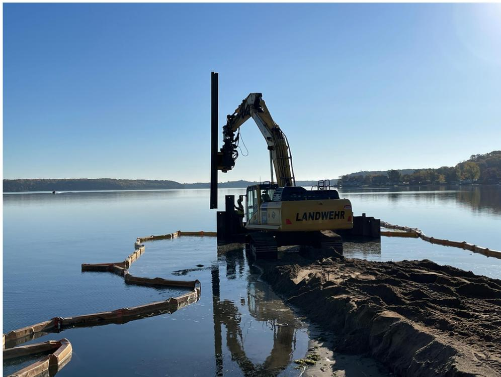
Photo #1: Installing Sheet Pile Wall for Inlet - Oct 16, 2023, 9:23 AM
