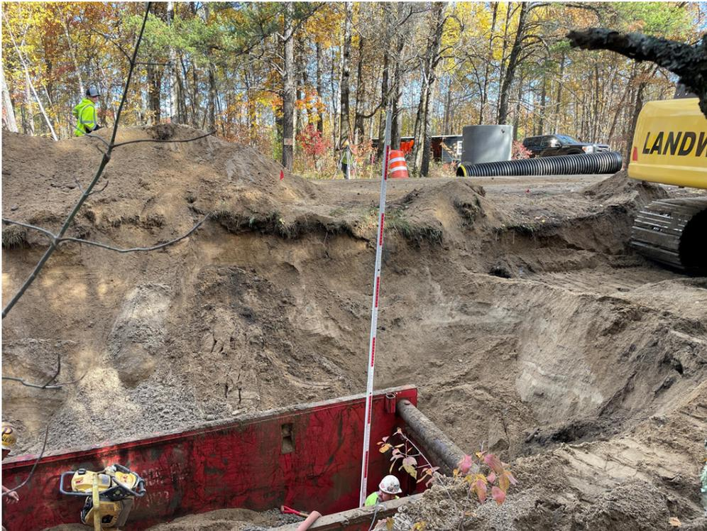
Photo #9: Measuring pipe elevation - Oct 20, 2023, 11:27 AM
