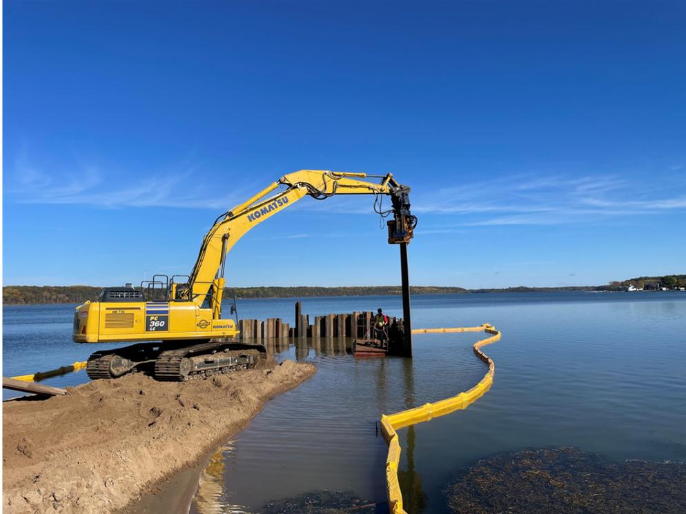
Photo #2: Sheet pile installation started along right side of causeway - Oct 17, 2023, 1:36 PM
