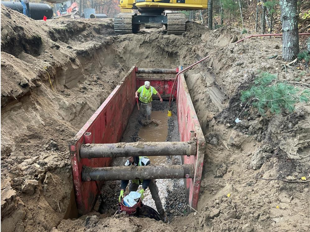
Photo #6: Leveling rock for gravity pipe to be placed on - Oct 20, 2023, 7:55 AM
