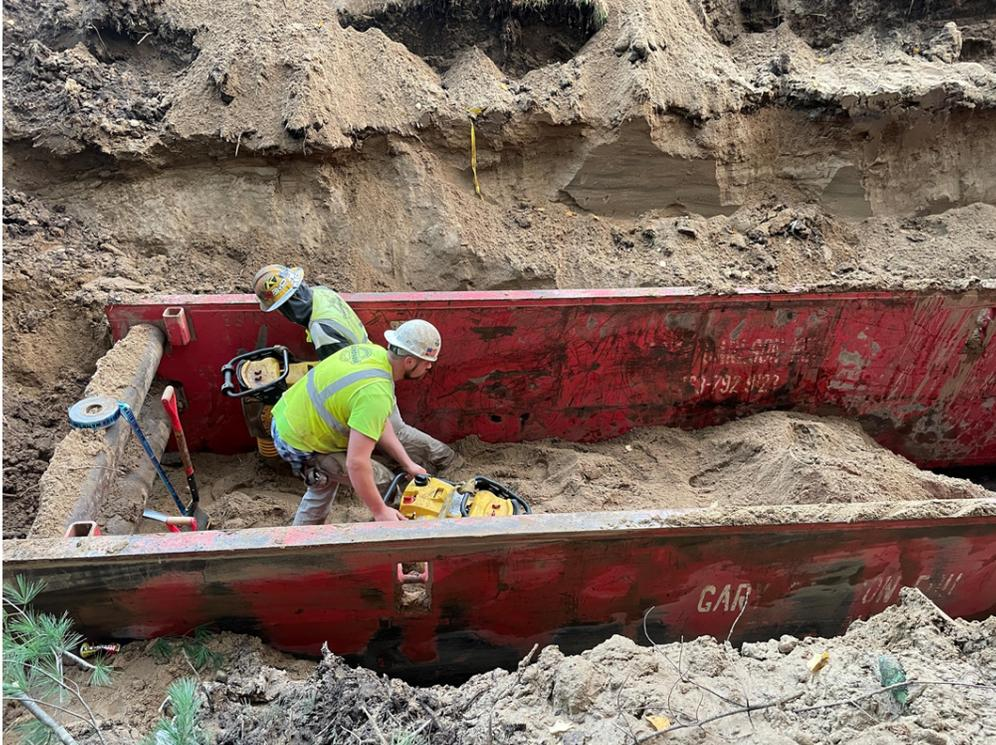
Photo #8: Packing sand in around pipe - Oct 20, 2023, 8:02 AM
