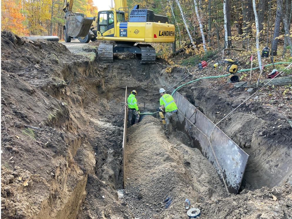
Photo #4: Packing sand around edges of pipe - Oct 19, 2023, 9:26 PM
