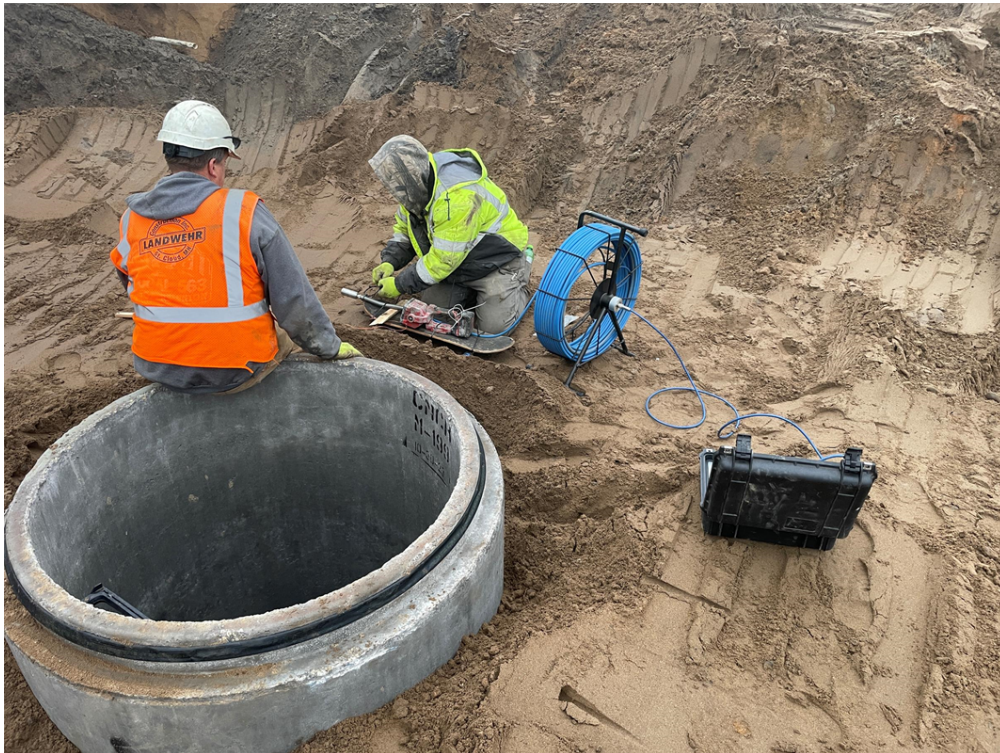
Photo #7: Preparing to televise gravity flow pipe - Dec 22, 2023, 8:37 AM
