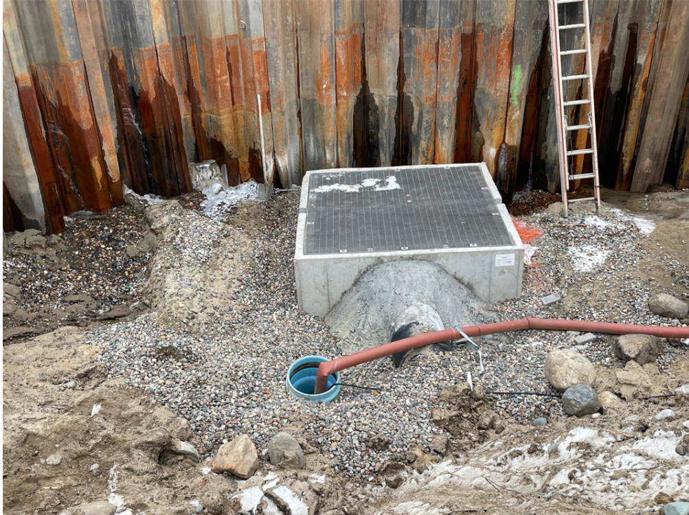
Photo #4: Inlet structure installed with screen - Dec 19, 2023, 3:10 PM
