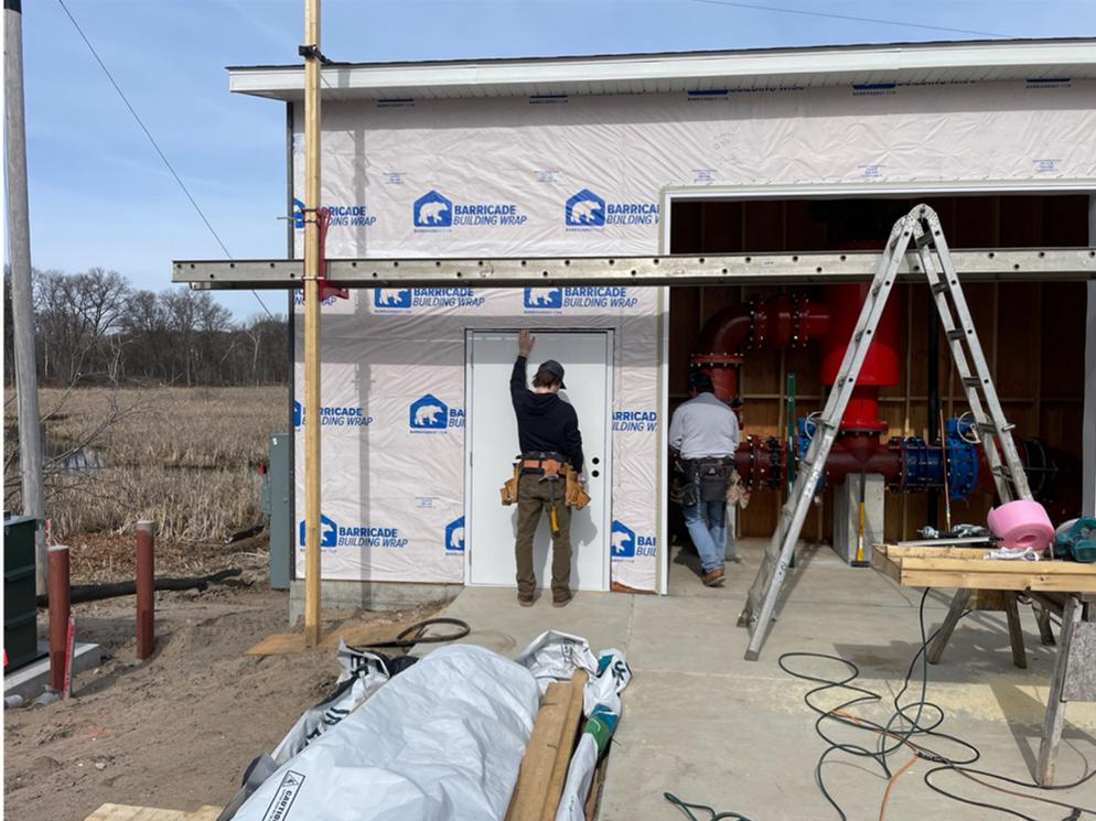
Photo #1: Installing the service door for the pump house - Apr 22, 2024, 10:02 AM
