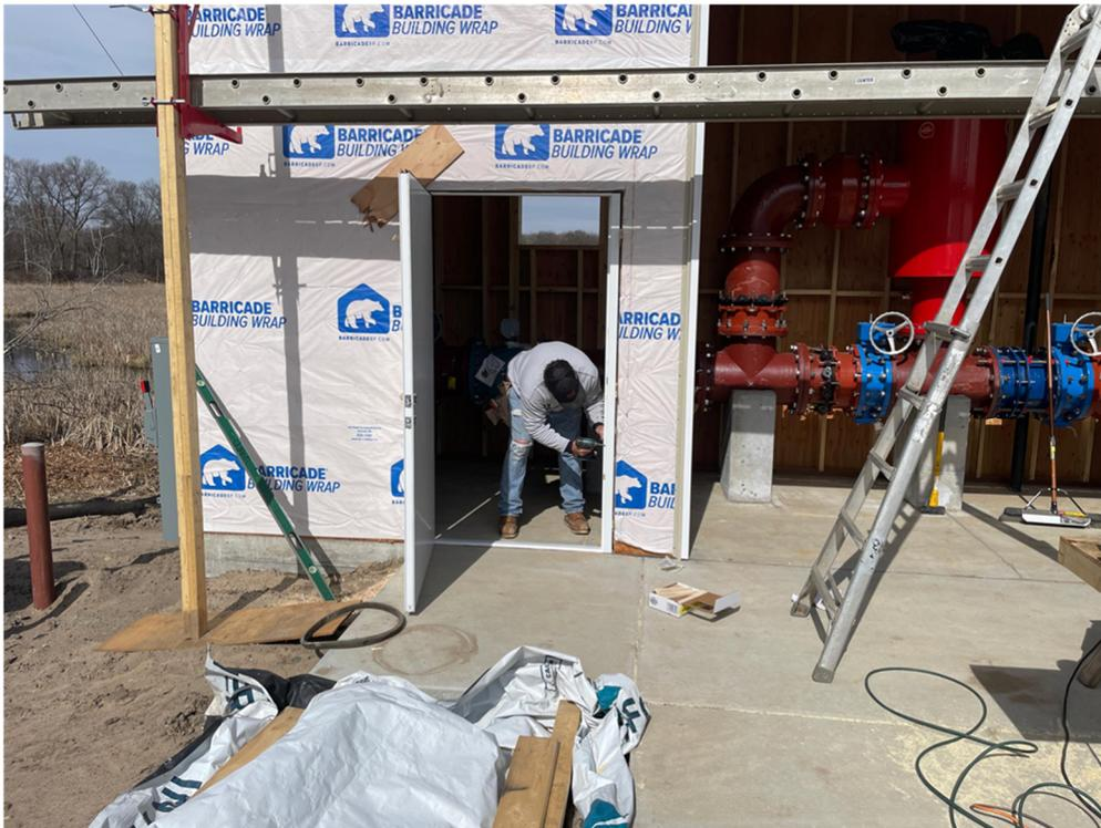
Photo #2: Attaching the door frame to the building framework - Apr 22, 2024, 10:27 AM
