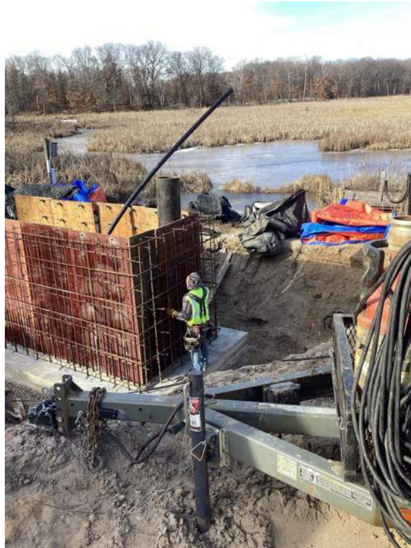
Photo #1: Installation of wall forms - Feb 19, 2024, 7:33 AM
