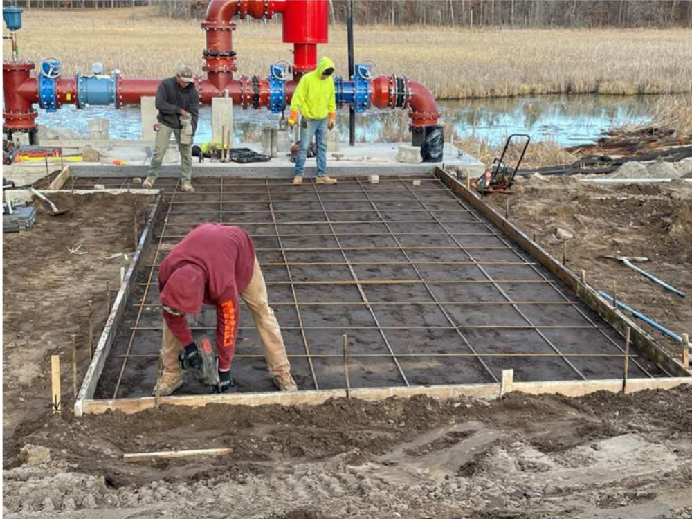
Photo #3: Setting and tying rebar within formwork - Mar 14, 2024, 8:47 AM
