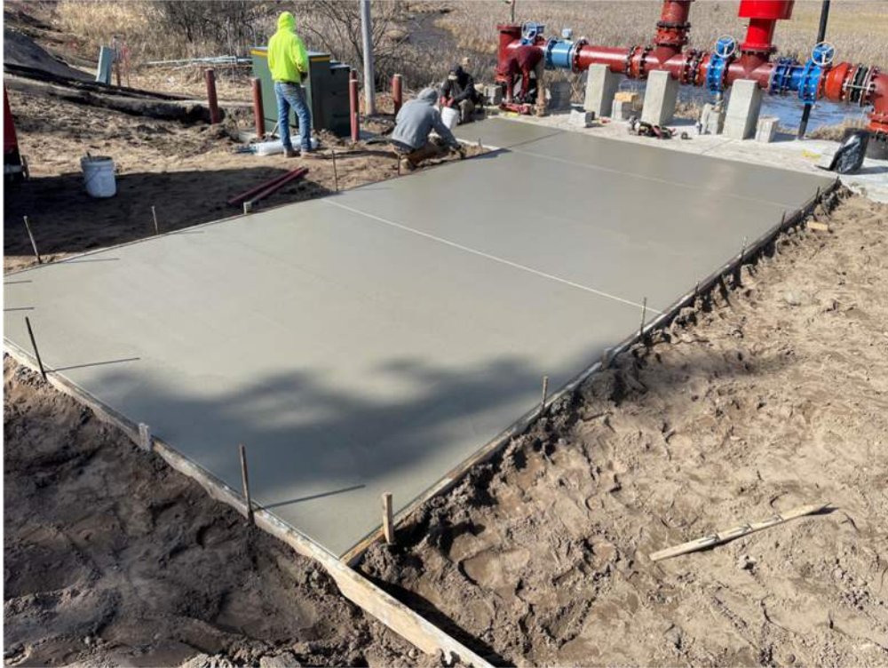
Photo #5: Concrete driveway in front of pump station - Mar 14, 2024, 11:26 AM
