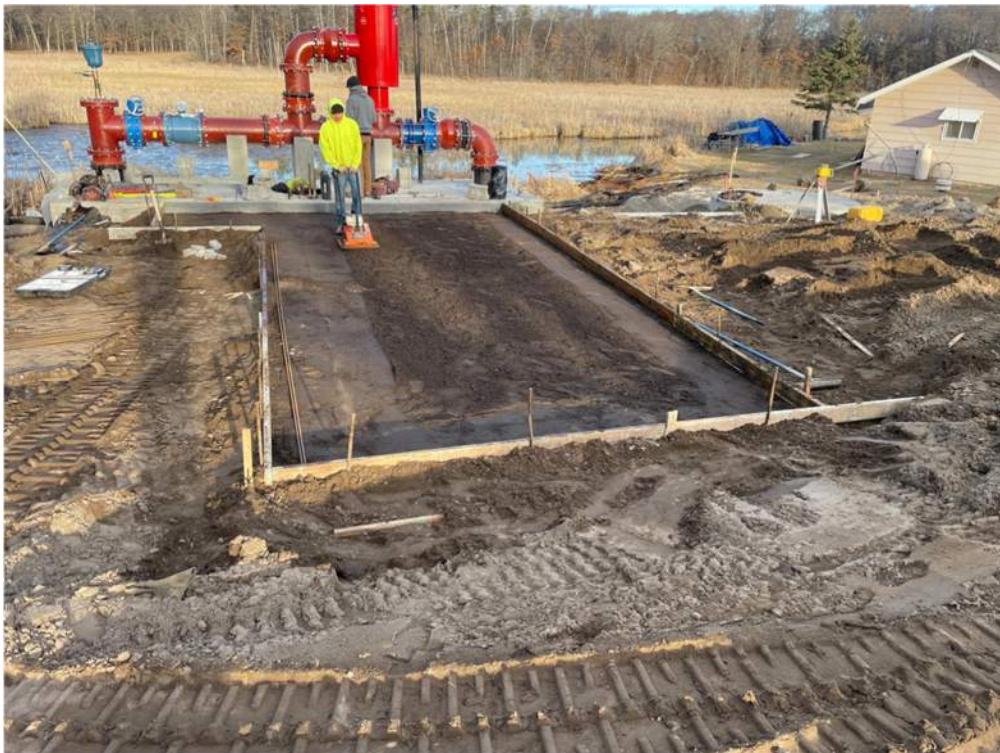
Photo #2: Form boards set for concrete driveway - Mar 14, 2024, 8:39 AM
