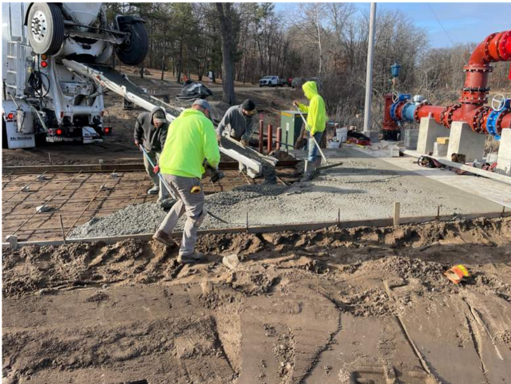
Photo #4: Pouring the concrete driveway for the pump station - Mar 14, 2024, 9:48 AM
