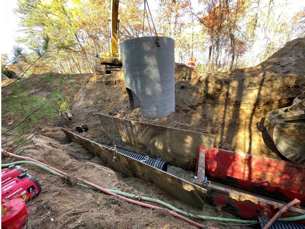
Photo #2: Installing manhole - Oct 23, 2023, 1:19 PM
