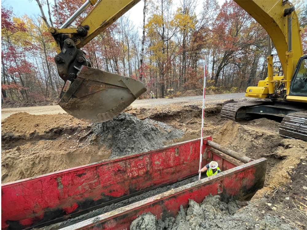
Photo #4: Checking pipe elevation - Oct 24, 2023, 10:43 AM
