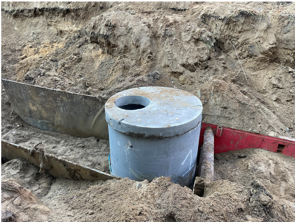
Photo #3: Top slab added to manhole - Oct 23, 2023, 4:14 PM
