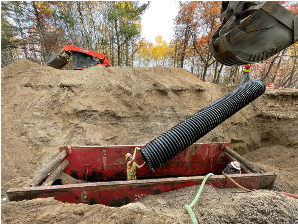
Photo #1: Installing 30" gravity flow pipe along Pulaski Road - Oct 23, 2023, 9:33 AM
