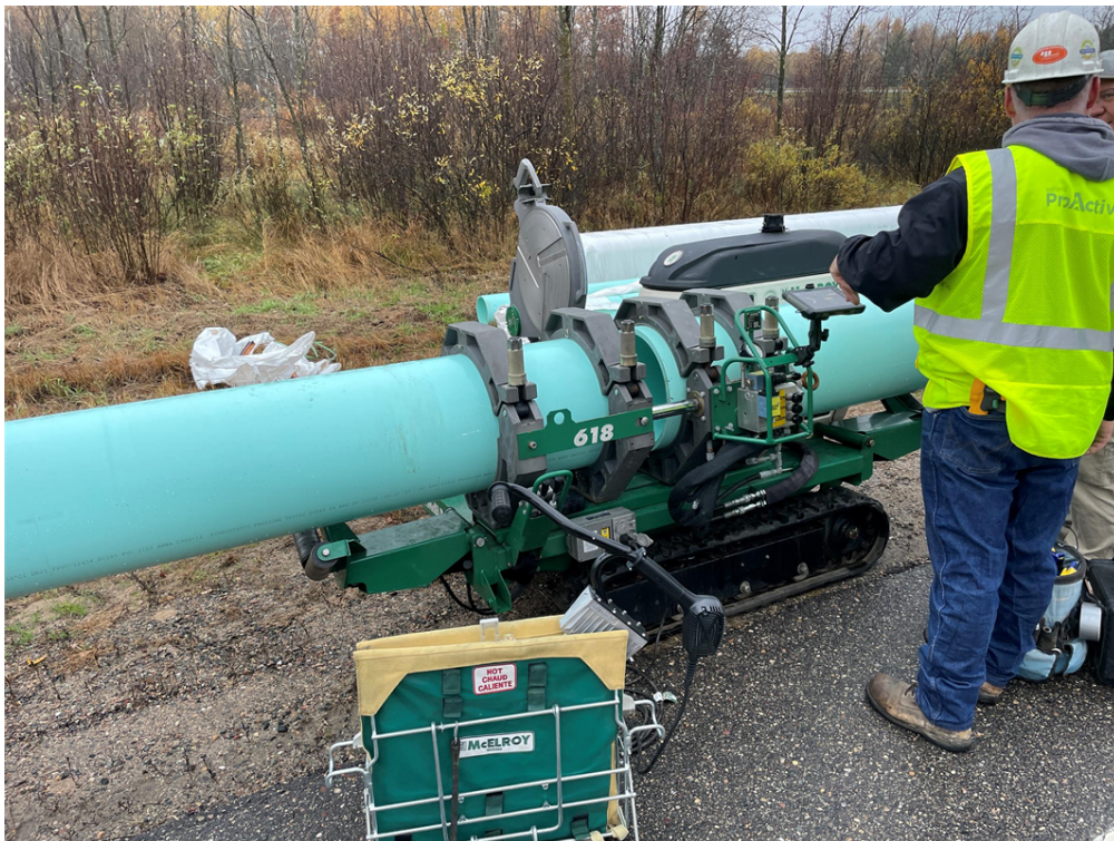
Photo #5: Preparing to fuse PVC pipe sections - Oct 26, 2023, 8:28 AM
