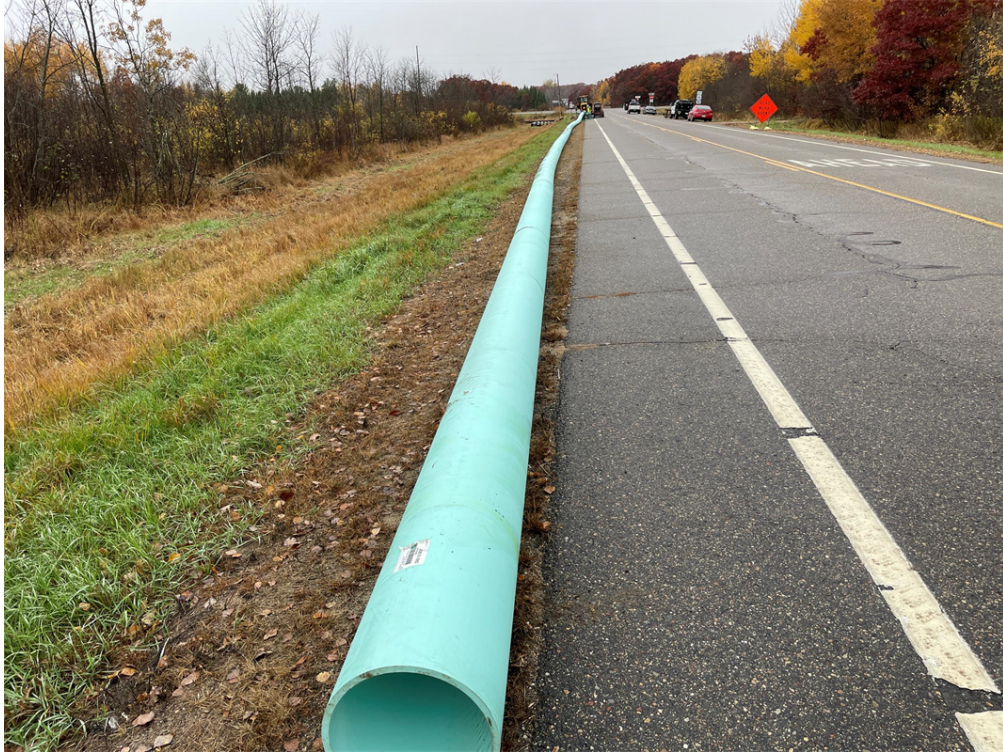
Photo #6: Fused 16" PVC pipe - Oct 26, 2023, 1:52 PM
