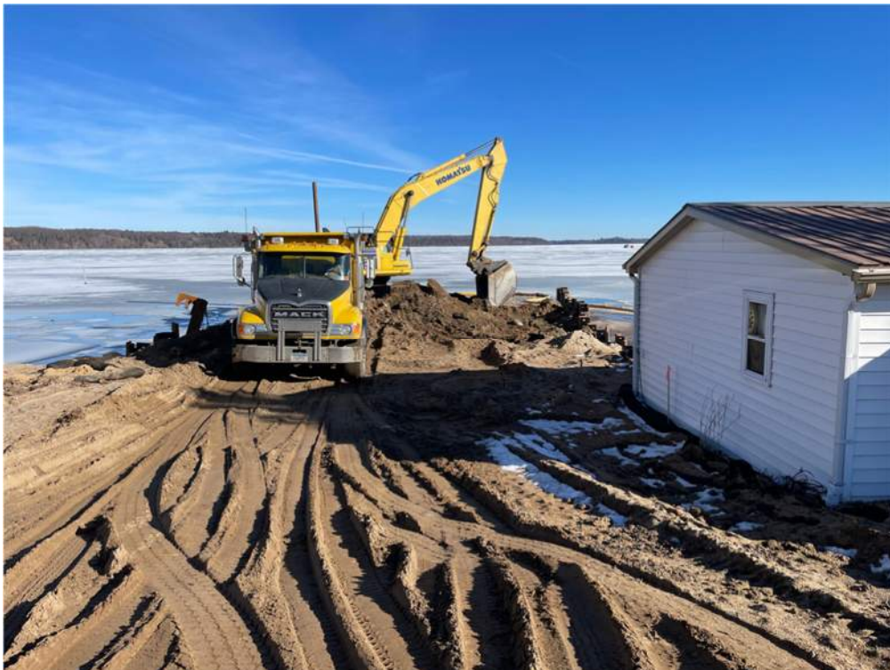
Photo #5: Removing sand from the cofferdam - Jan 31, 2024, 1:34 PM
