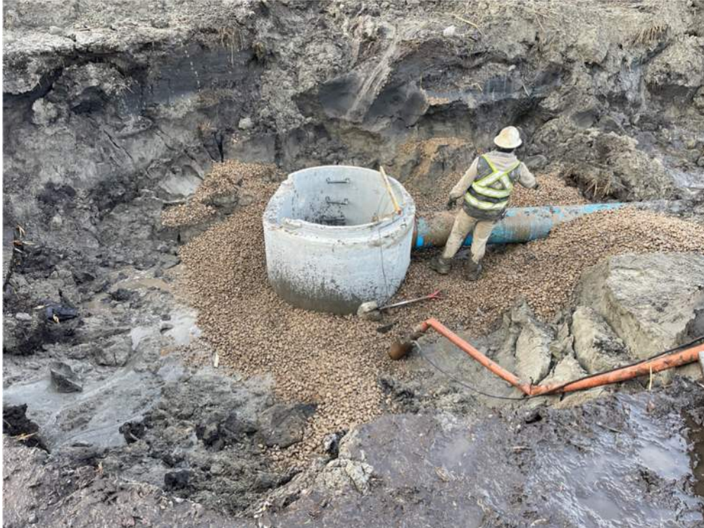
Photo #4: Force main outlet structure base section set - Jan 30, 2024, 4:17 PM
