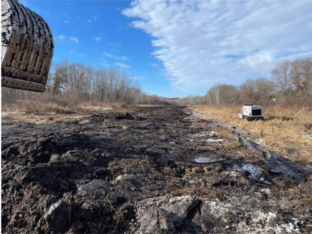
Photo #2: Backfilling soil over pipe - Jan 29, 2024, 10:37 AM
