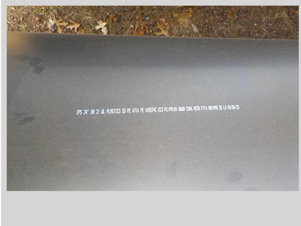
Photo #6: 24" Dia inlet piping - Oct 12, 2023, 11:21 AM
