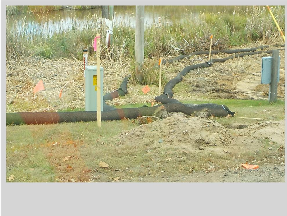
Photo #1: Double Stack Bio-roll - Oct 11, 2023, 12:55 PM
