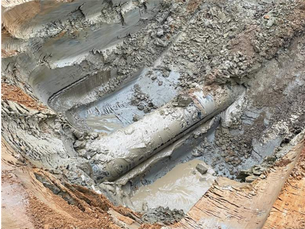
Photo #1: Bored carrier pipe going under County Road 203 - Nov 6, 2023, 7:44 AM
