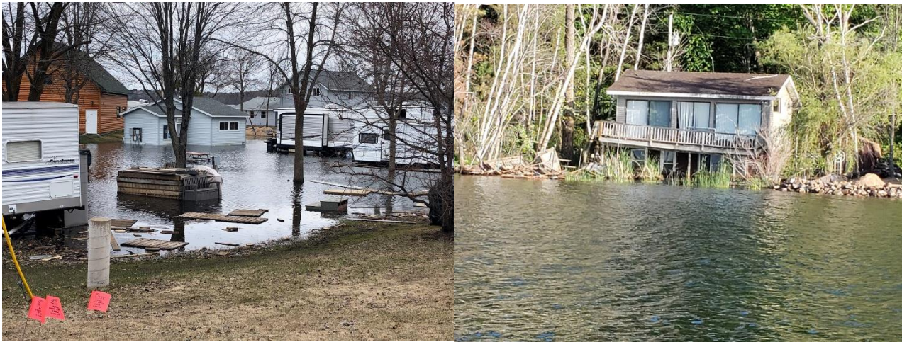
Example of flooding at Augers Resort and destroyed cabin.
