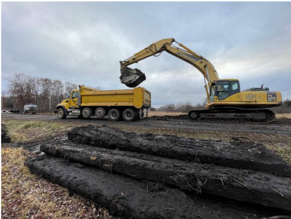
Photo #3: Loading excess material to haul offsite - Nov 21, 2023, 9:19 AM
