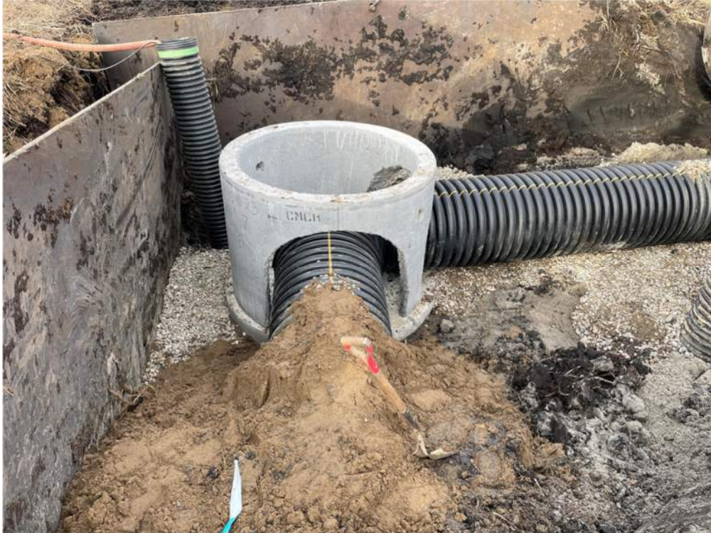
Photo #2: Gravity flow pipes installed inside of manhole 7 - Nov 20, 2023, 2:24 PM
