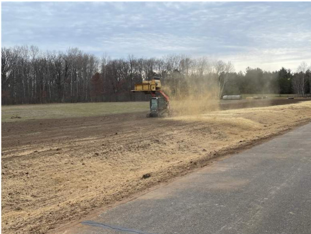
Photo #7: Spreading straw over seeded field - Nov 22, 2023, 12:40 PM
