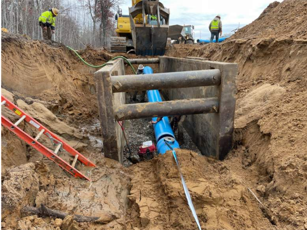
Photo #8: Installing force main pipe along Highway 10 headed South - Nov 22, 2023, 1:10 PM
