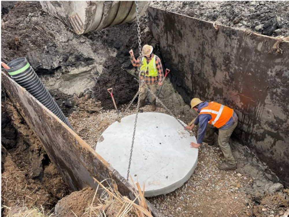
Photo #1: Installing base slab for manhole 7 along Atlantic Road - Nov 20, 2023, 11:38 AM
