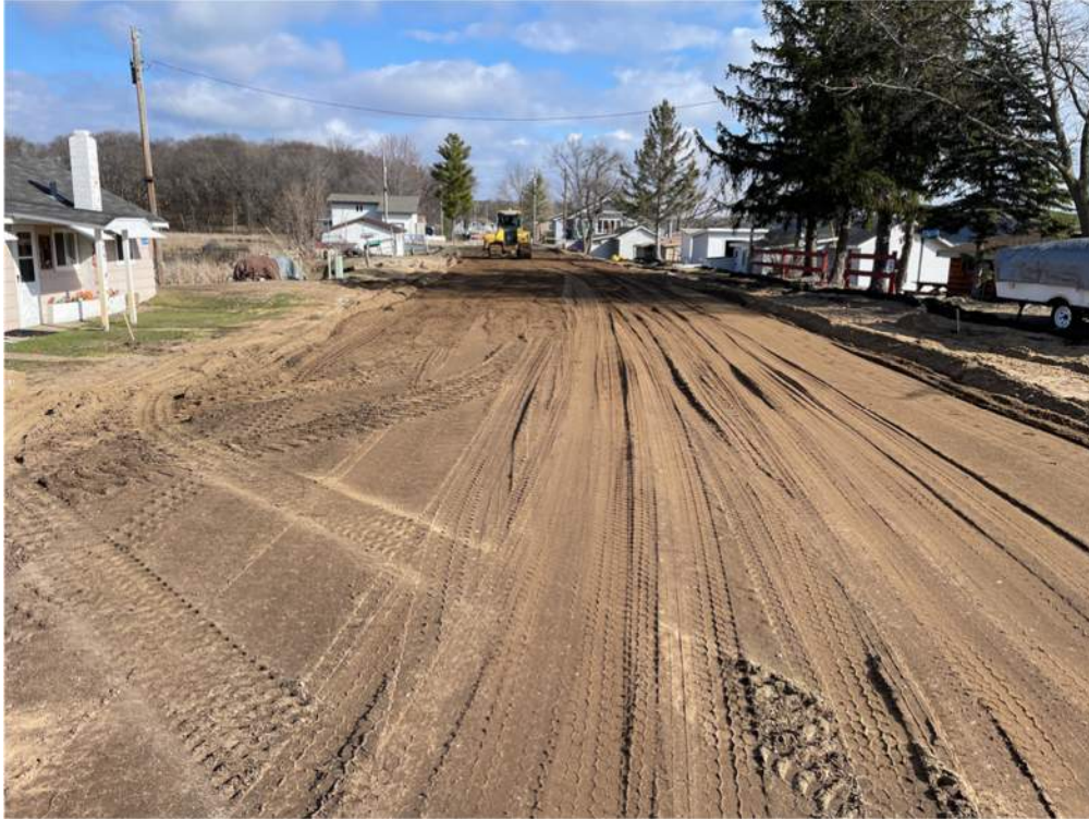
Photo #7: Spreading gravel base on Aztec Road - Apr 11, 2024, 9:42 AM
